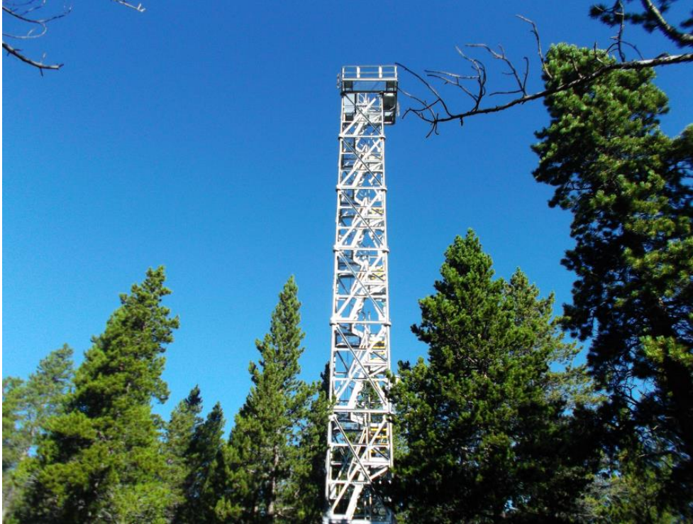
Figure 1. Comparable tower built in Rocky Mountain National Park
