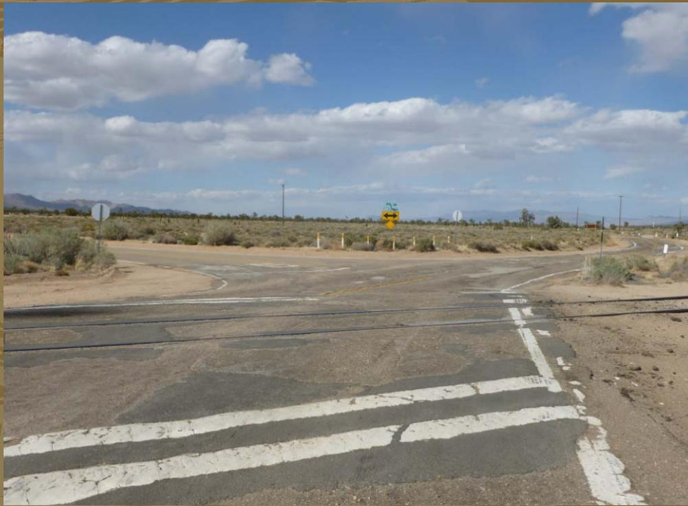
Problem: A railroad spur line on Kelso-Cima is 5-7 feet above the road grade, resulting very limited sight distance. Further, after crossing the tracks from the south, drivers are faced with these three roads forming a very confusing Y intersection. This results in rear end collisions and cars driving off the road.
