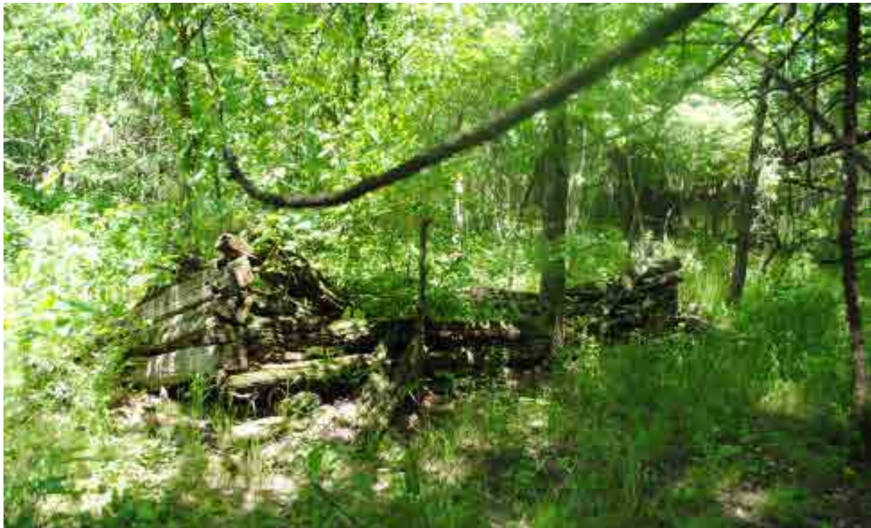
Figure 3-54. The remnant log cabin in Morgan's Woods to the west of Lee Creek is a brick foundation with hand-hewn, squared log timbers with dove-tail joints. The cabin measures twenty-feet by sixteen-feet (MB: DSC_0273.jpg).
