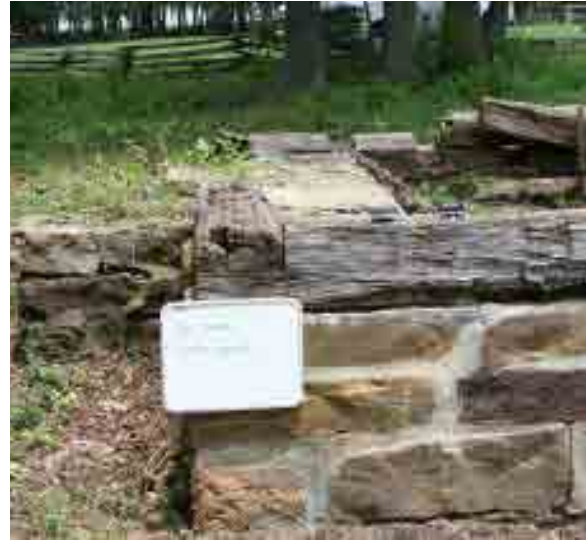
Figure 3-52. The Winton Springs House was demolished in the 1990s after recommendations for its removal were made. The foundation remains, including hand-hewn timbers set on a flagstone base (MB: IMG_4237.jpg).
