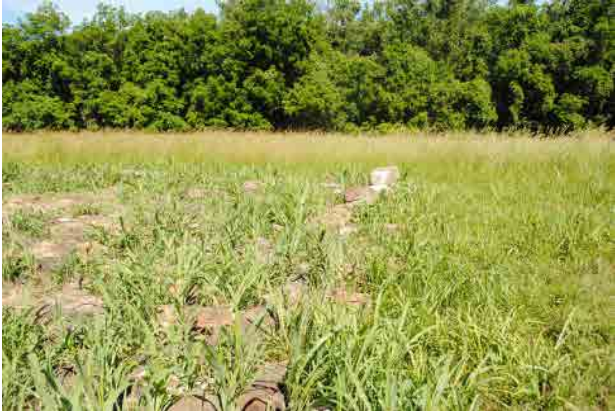
Figure 3-55. A house foundation near tour stop 2 consists of stone blocks, and measures approximately twenty-feet square. The foundation is covered with grasses and is in good condition (MB: DSC_0089.jpg).
