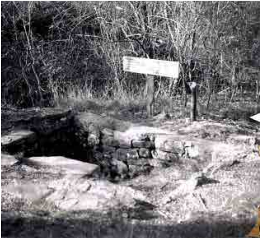
Figure 3-143. The spring box at Elkhorn Tavern is built of stone, and is approximately eight-feet square (5-04-67 trail to spring.tif).
