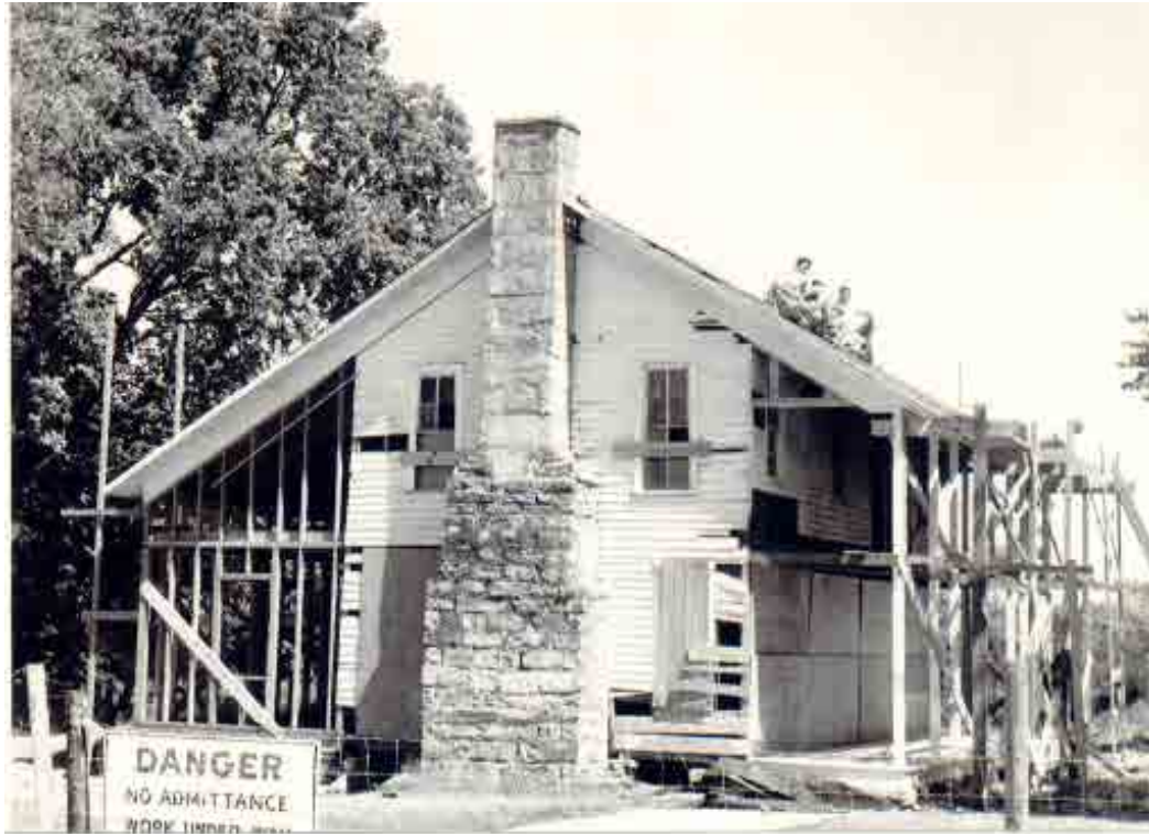
Figure 3-135. Elkhorn Tavern was rebuilt in the 1960s to reflect to its 1880s appearance. Work included removing the rear (west) extension and modifying the double porch at the building's front facade (B&W Southeast corner under restoration.jpg).
