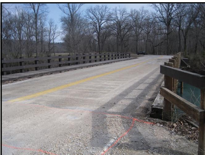
The timber bridge deck is covered with asphalt pavement. Water drains through the asphalt and becomes trapped against the timber deck surface, promoting decay.
