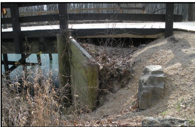
There has been a loss of backfill material at the north and south abutments. The loss of backfill creates sinkholes in the approach roadways.
