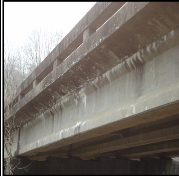
Figure 1b: Efflorescence buildup
