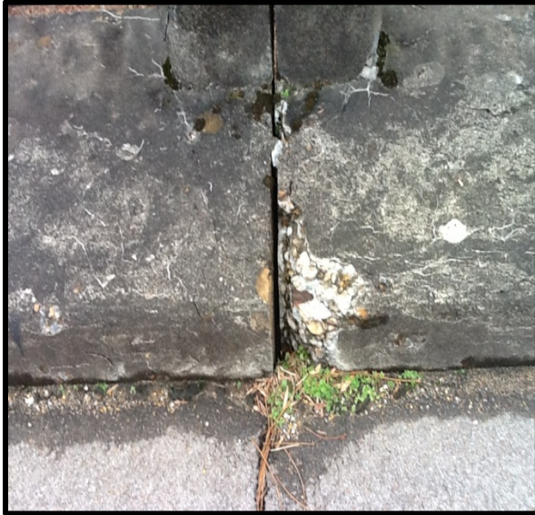
Figure 1a: Delamination of pier caps
