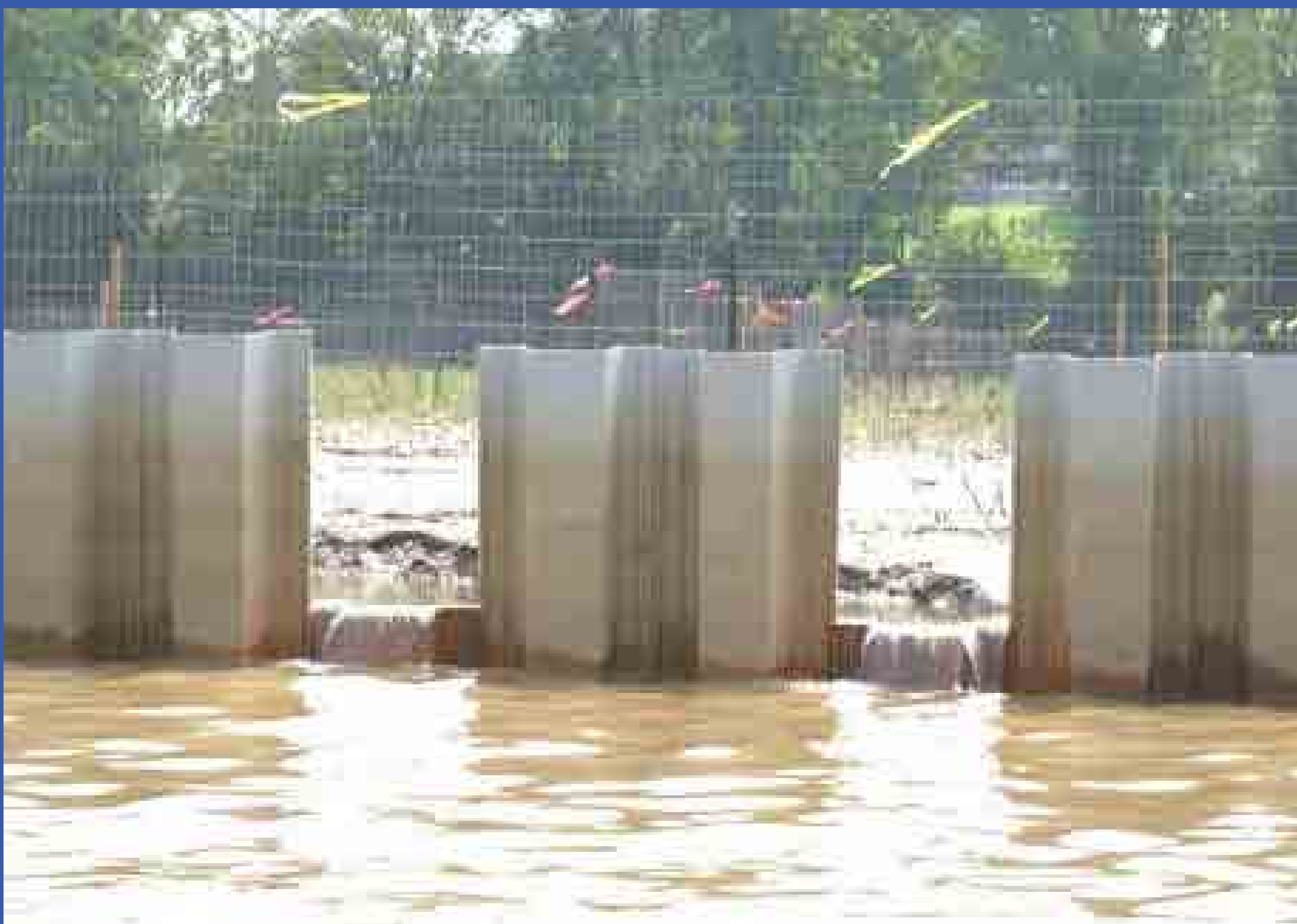
Example of sheet piling configured to allow for intertidal exchange.
