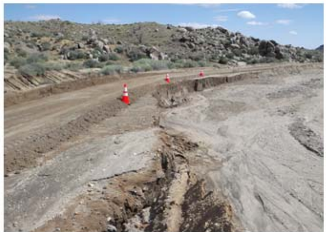
Black Canyon Road Slope Protection
