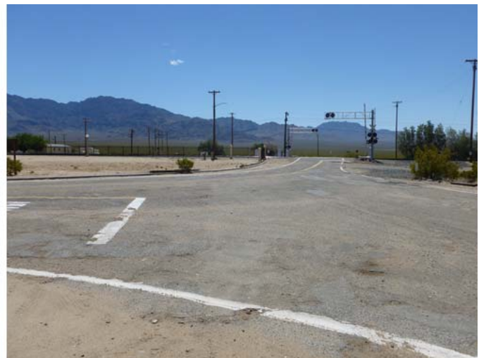
Photo showing limited sight distance at railroad crossing
