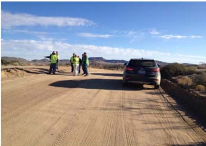
Black Canyon Road Curve Improvement Site
