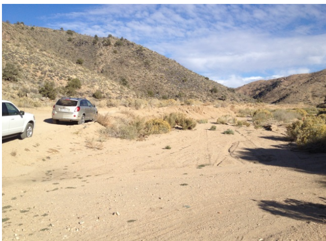
Photo Showing Low Water Crossing on Cedar Canyon Road
