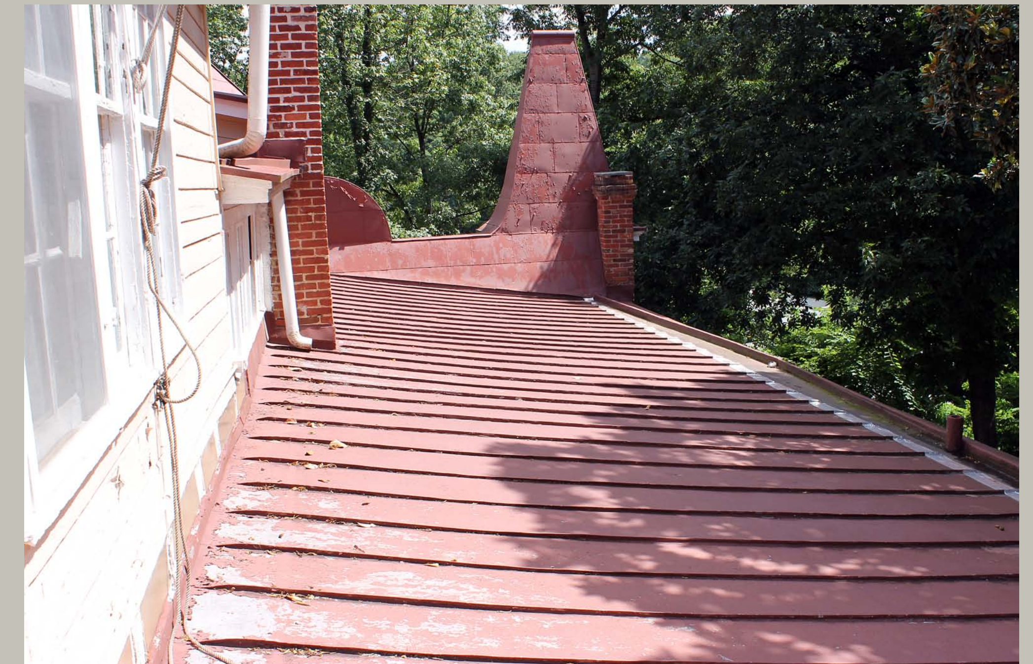
LOW SLOPED METAL ROOF SEGMENTS WITH GUTTER TAPE ON THE EDGES.
