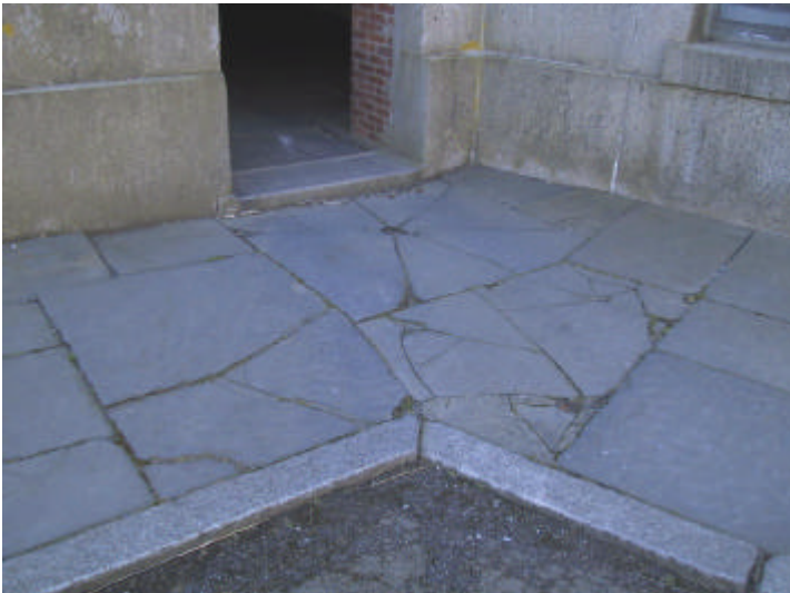
Figure 6 – Badly cracked bluestone pavers in Bastion D
