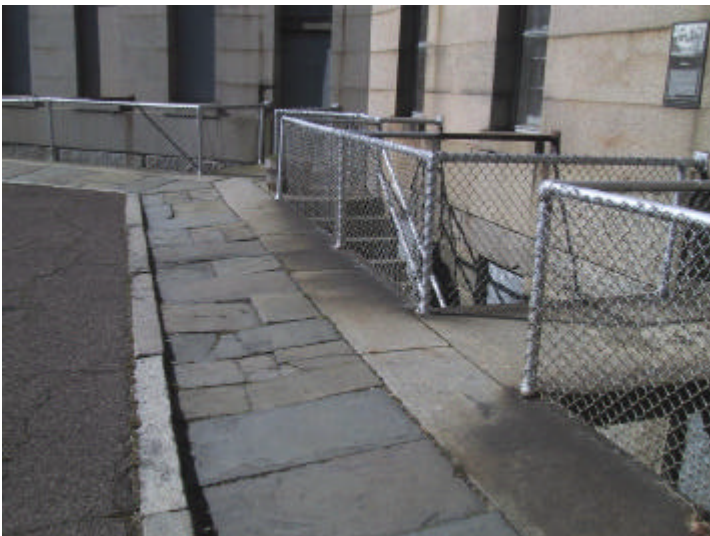
Figure 7 – Bluestone pavers and granite curbs badly misaligned in Bastion C.
