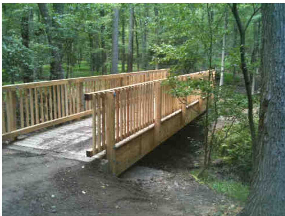
FIGURE 5. EXAMPLE OF ENWOOD© LAMINATED WOOD BRIDGE
