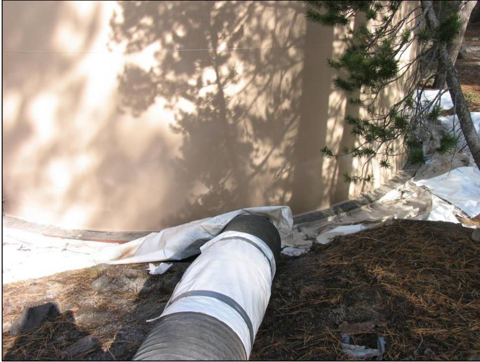
Photograph 5: Negative Air Flow Tubing (NPS Photos 2005)
