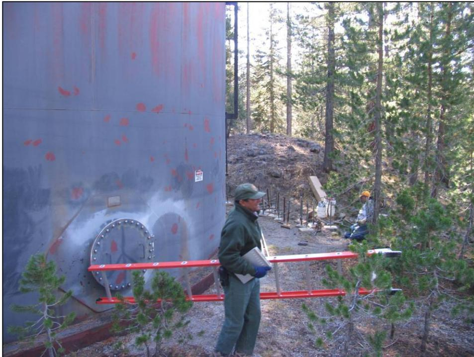
Photograph 2: Water Tank and Weathered Paint (NPS Photos 2005)
