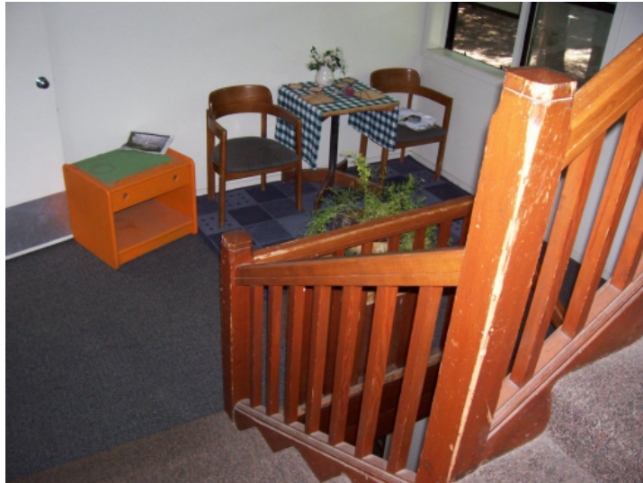
Figure 2: Door Blocked Open, Combustibles in Stairway Enclosure in Tecoya E
