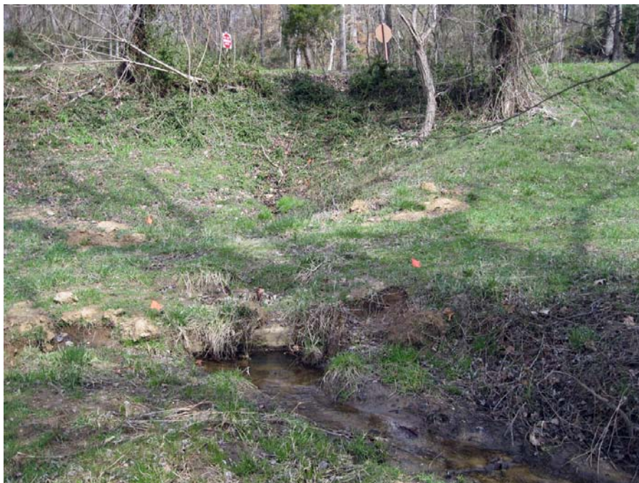
View of the far southern culvert. The culvert has collapsed and under the proposed project it and the headwalls will be replaced.
