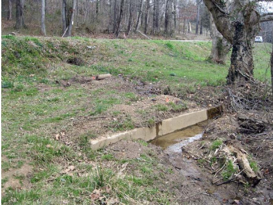
View of one of the middle culverts. The culvert has collapsed and under the proposed project it and the headwalls will be replaced.
