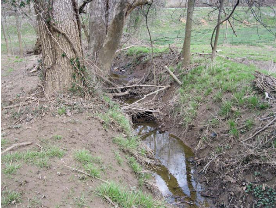
View of the southern drainage ditch. Note the debris and vegetation growth. Under the proposed project the ditches will be cleaned and cleared.
