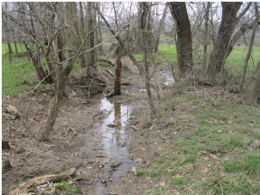
View of one of the middle drainage ditches. Note the debris and vegetation growth. Under the proposed project the ditches will be cleaned and cleared.
