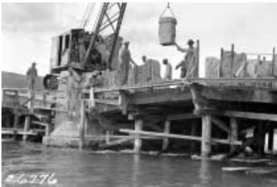
St. Mary Bridge under construction, showing ring stone being placed
