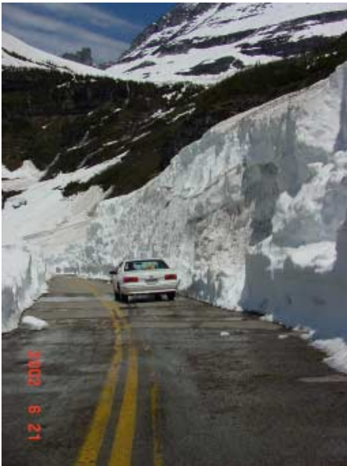
Overhanging snow on the Going-to-the-Sun Road
