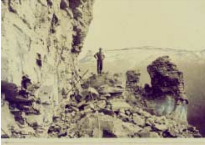
Original road construction
