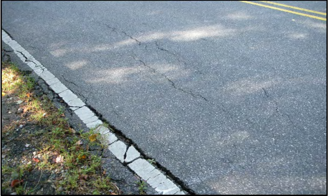
Figure 9. Roadway cracking and settling
