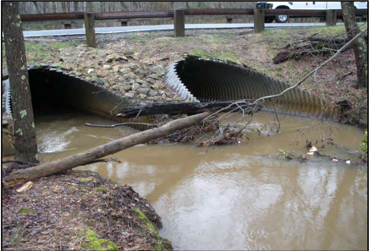
Figure 1. Corroded double culverts at Still Creek (upstream)
