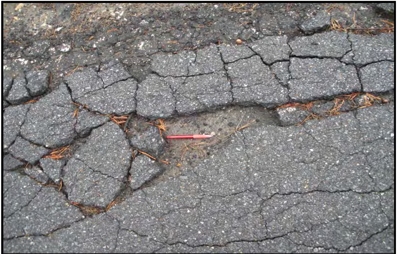
Figure 10. Edge of pavement cracking
