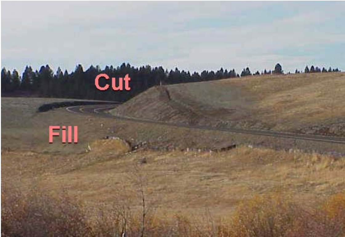
Figure 2.3 – Example fill to the left of the roadway and cut to the right of the roadway. Both exceed 40 feet in height
