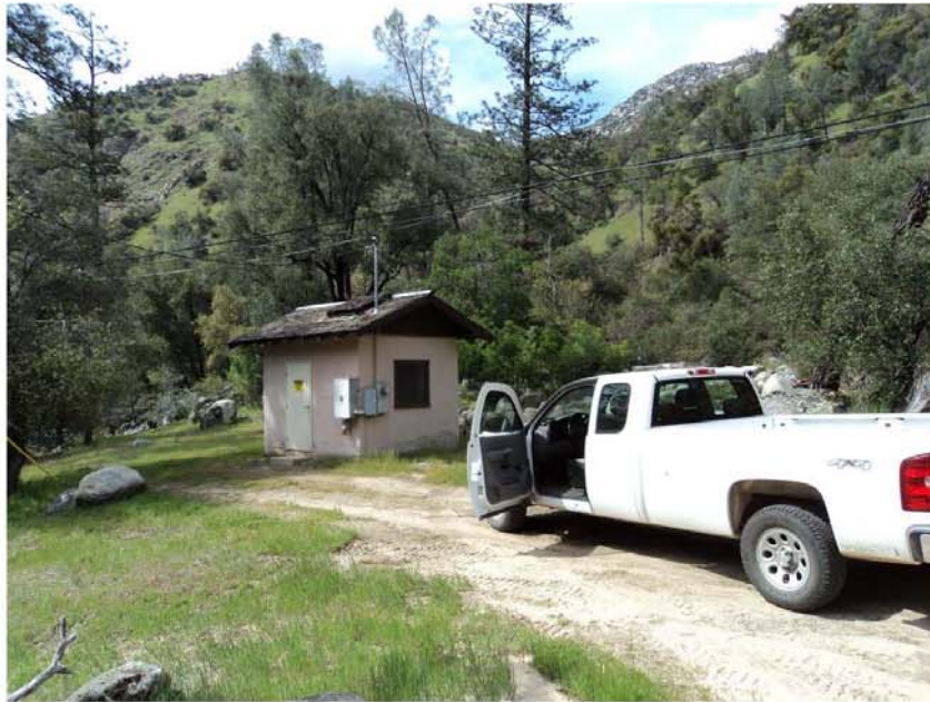
EP Well House #2
