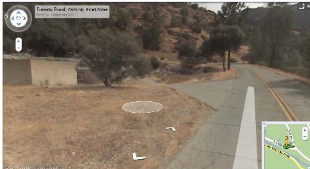
Below picture shows the El Portal Wastewater Treatment Plant on Foresta Road. The intersection of Spur Road and Foresta Road is in the background.
