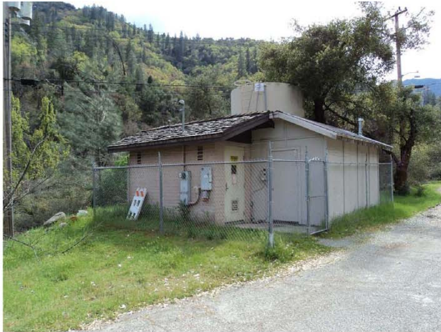
EP Well House #4
