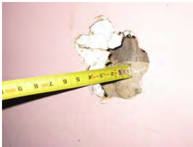
Figure 2-044: Gypsum wall board furled out at room 109 south wall. (Photo: BBB, 2006)
