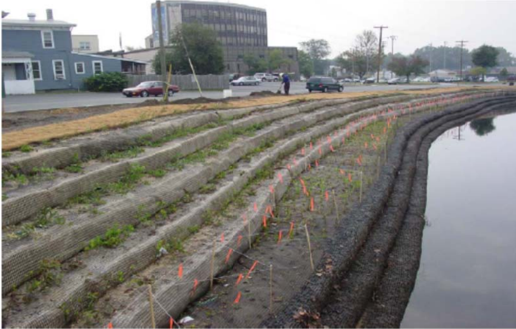
FIGURE 2-6: EXAMPLE OF VRSS AFTER CONSTRUCTION
