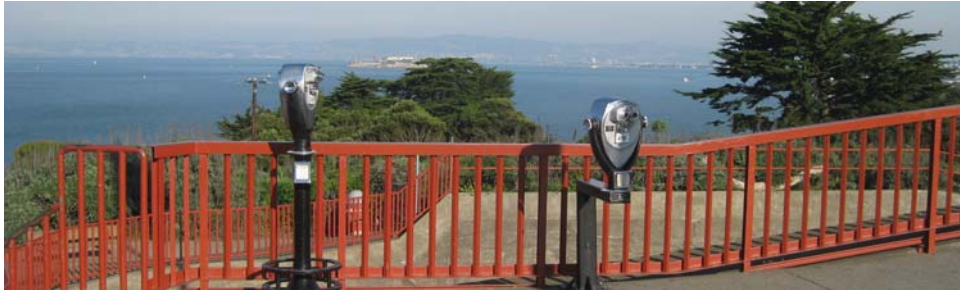
The Golden Gate Bridge south access area has open views, is limited in size and very congested
