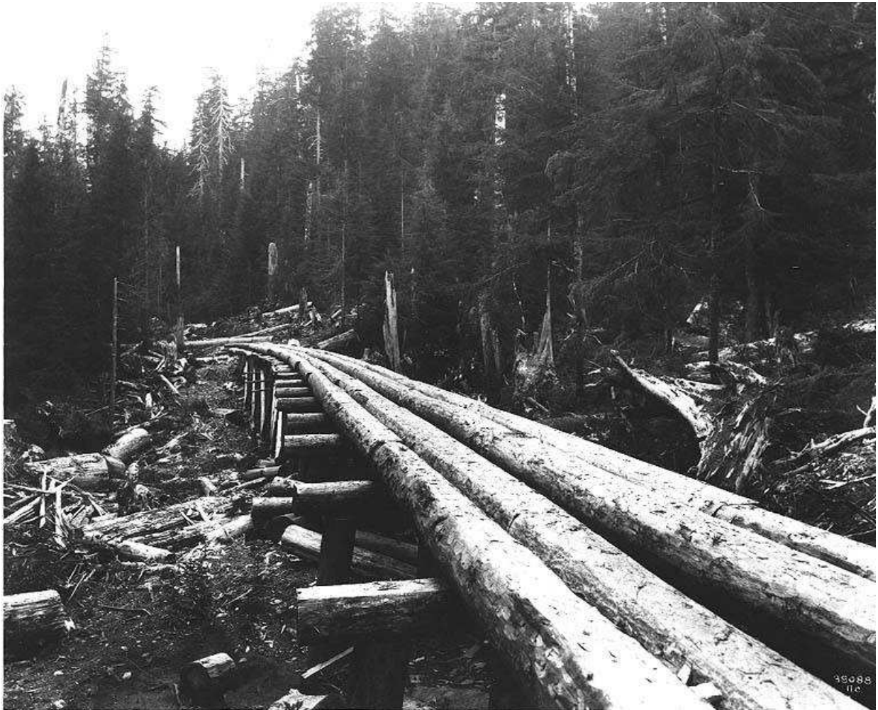
Figure 20. “Log railroad bridge under construction, U. S. Army Signal Corps Railroad, Spruce Production Division, Lake Crescent area.” Asahel Curtis Photo Collection (PH Coll. 482,
