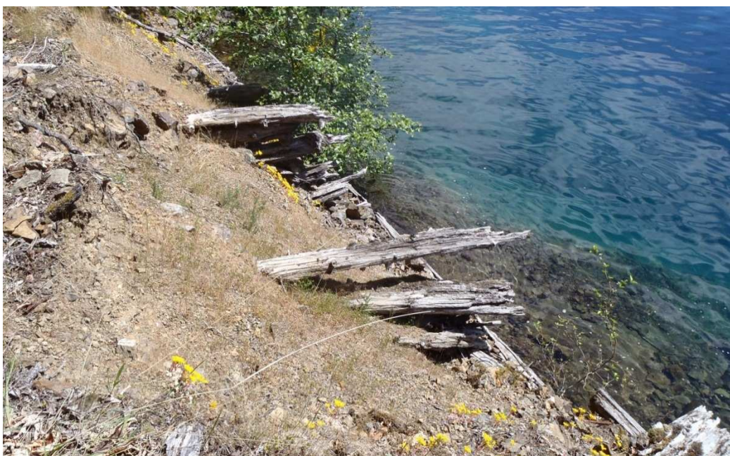
Figure 26. Timber half-bridge remains, mile 1.98 (Wray 2011)
