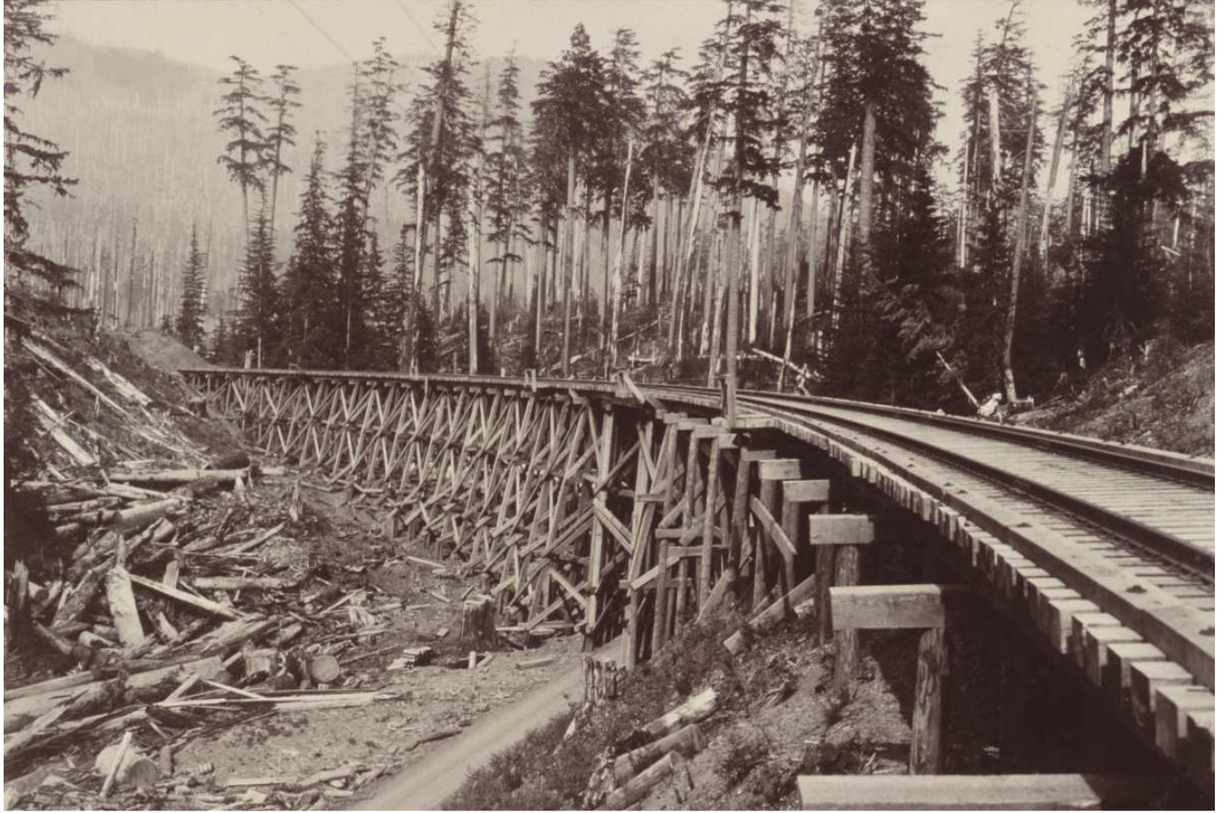
Figure 27. Sol Duc area (falsework)
