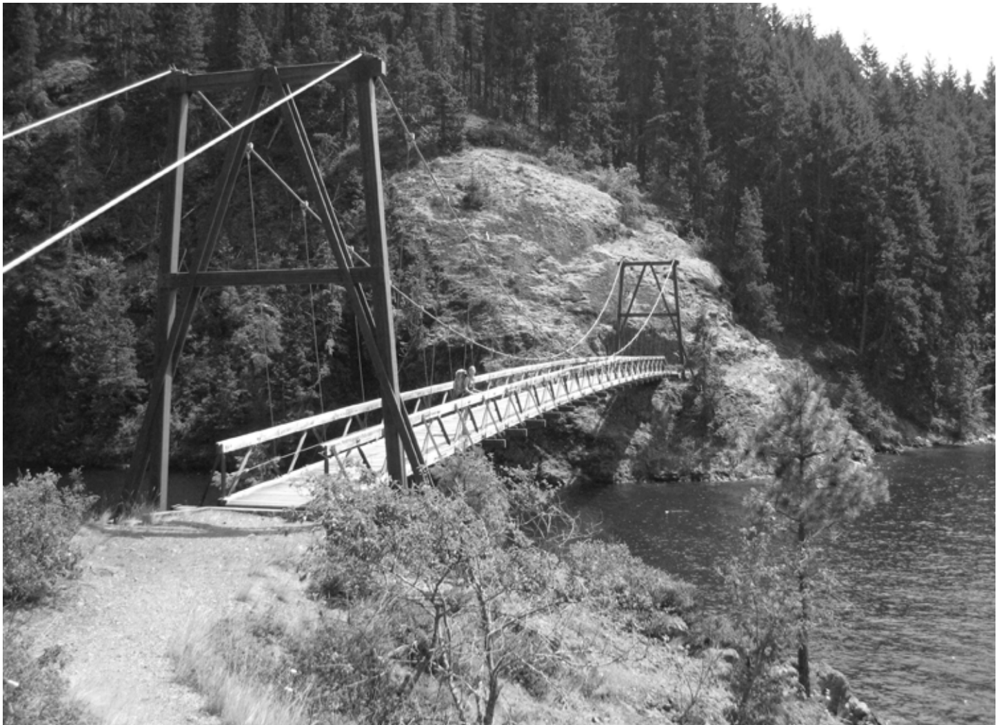
Bridge over Lightning Creek.
