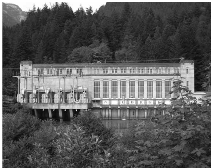
Seattle City Light's hydroelectric facilities have a long history in the upper Skagit River basin.
