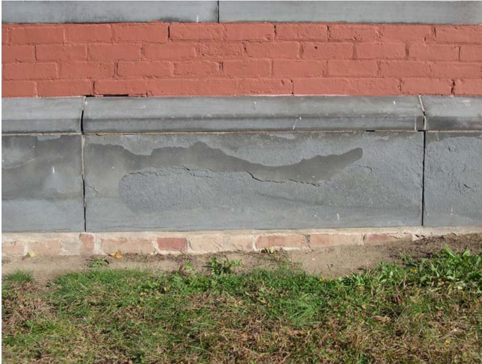
Exterior 5. Spalling bluestone water table and open mortar joints at the northwest corner of the 1905 north wing addition (JGWA 2008)
