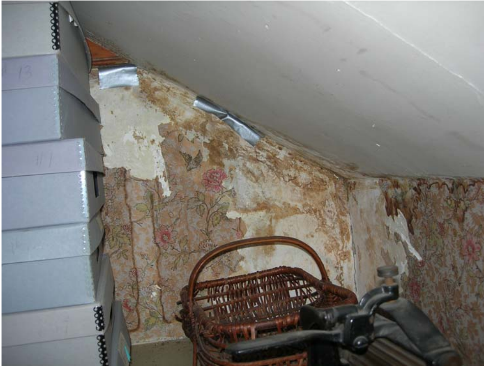
Interior 4. Room 213, “Alice’s Bedroom Closet”, exhibits extensive water damage and plaster deterioration along the northeast exterior wall (JGWA 2008)
