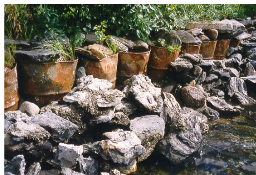
Photograph 2: Close-up of Retaining Wall
