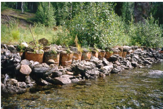
Photograph 1: Walker Lake Retaining Wall
