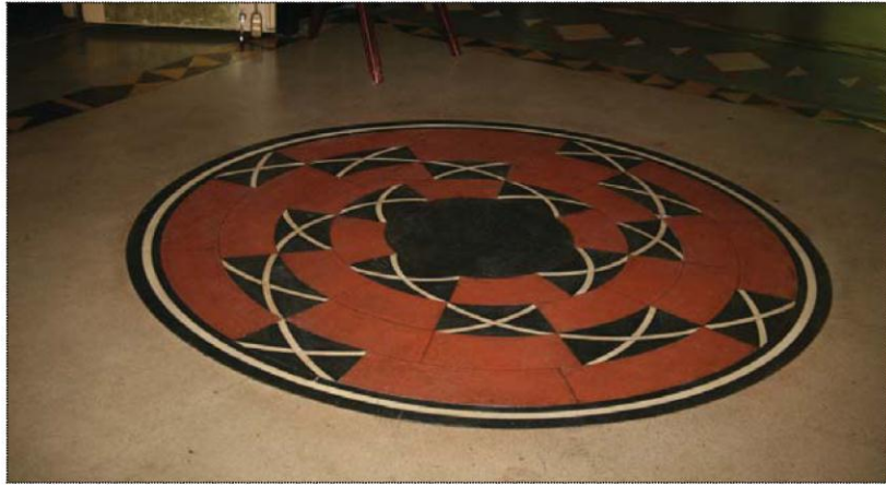
Figure 252: Detail view of the Registration Lobby rubber floor tiles, 2009. (Source: ARG)
