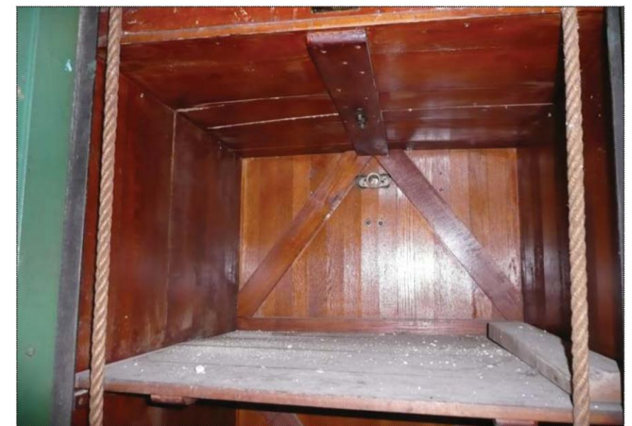
Figure 262: Detail view of dumbwaiter in Basement, 2009. (Source: ARG)
