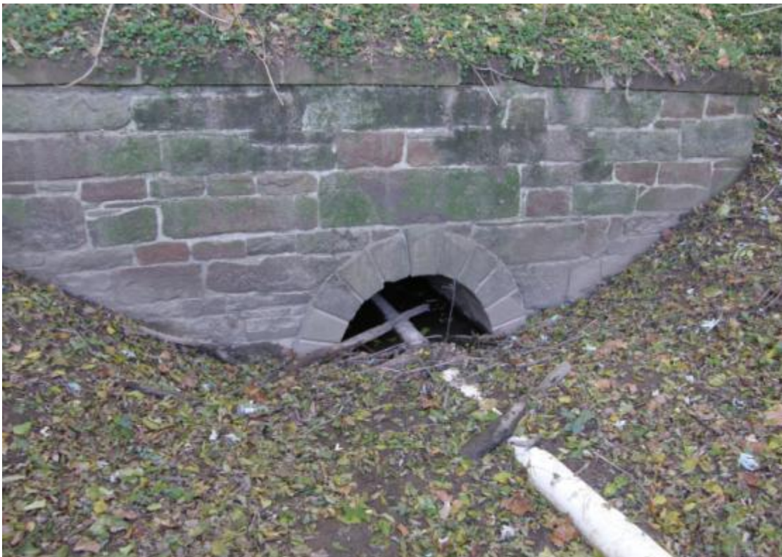
Figure 6. View of Culvert #39, Showing Existing Water Intake Line
