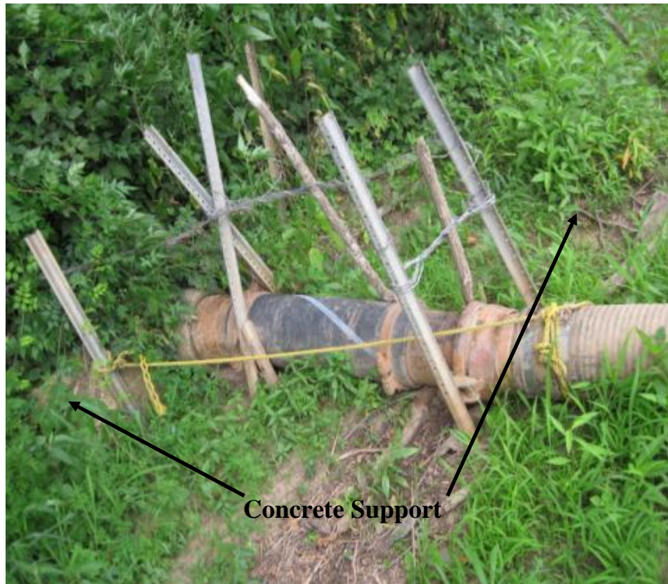
Figure 3. Existing Line #1 Anchored on the Shoreline
