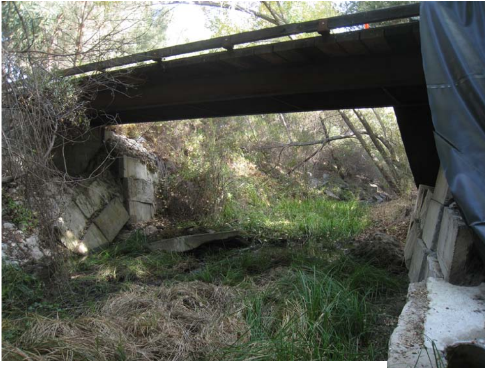
Figure 12: Damaged bridge and old abutments to be removed.
