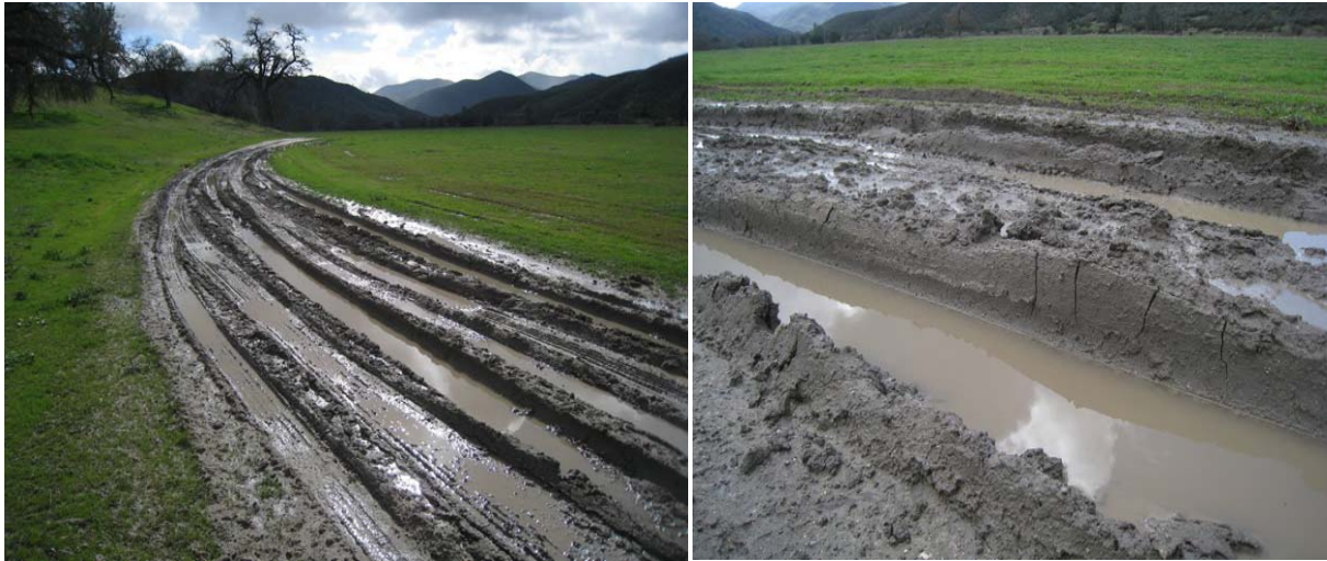
Figure 23: Access to the Historic District from Highway 25. Soil and vegetation damage is evident in the development of ruts and parallel tracks that occurs during wet conditions. When not wet, this is a source of airborne dust.
