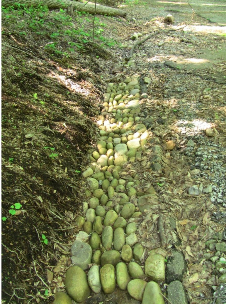
Figure 13: Historic Cobble Stone Gutter
