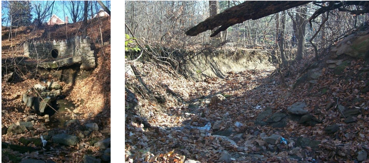
Figure 1: Storm water Damage in Fairmount Park, Pennsylvania (before)
