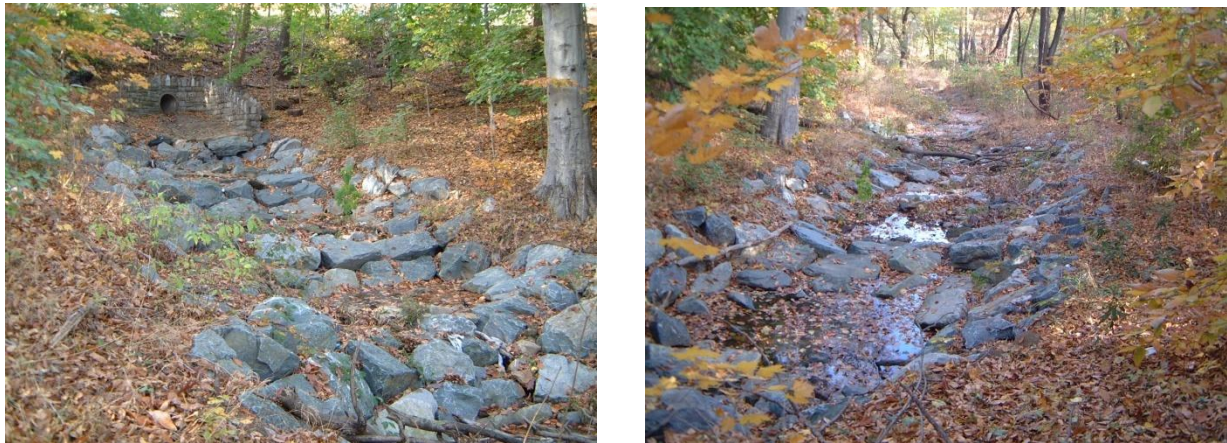
Figure 2: Installed RSC in Fairmount Park, Pennsylvania (after)
