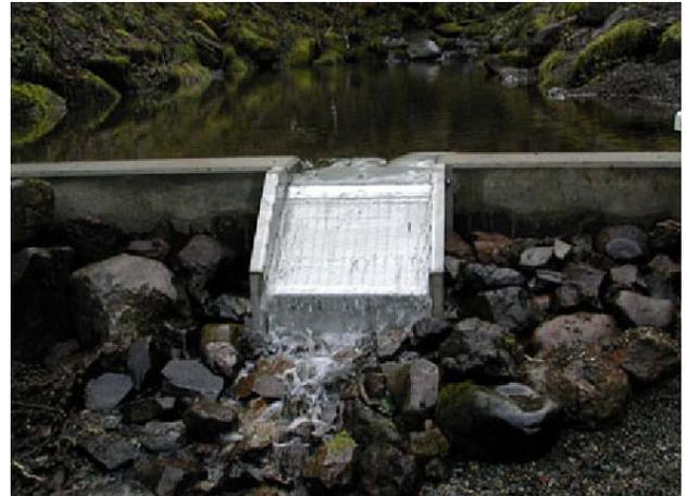
**Photo 13. Example photo of a wedgewire screen water intake structure** (photo courtesy of [www.hydroscreen.com](http://www.hydroscreen.com)).
