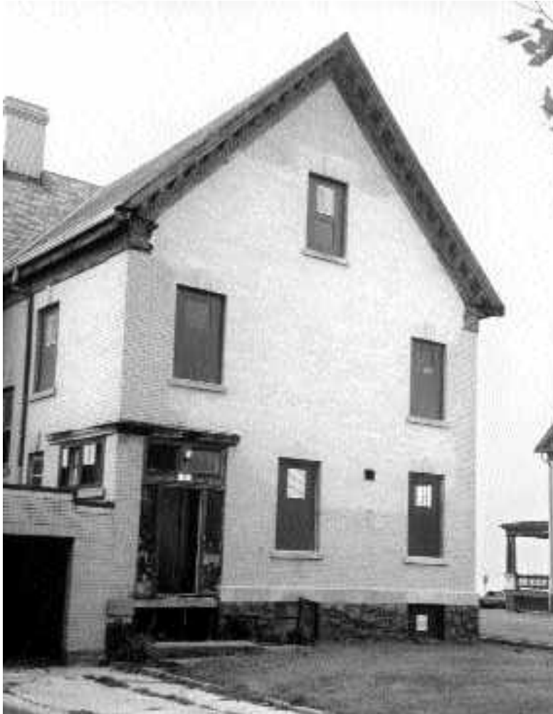
East wall of Building 10, which was rebuilt using new anchoring system, new brick and replacement steel in lintels.
