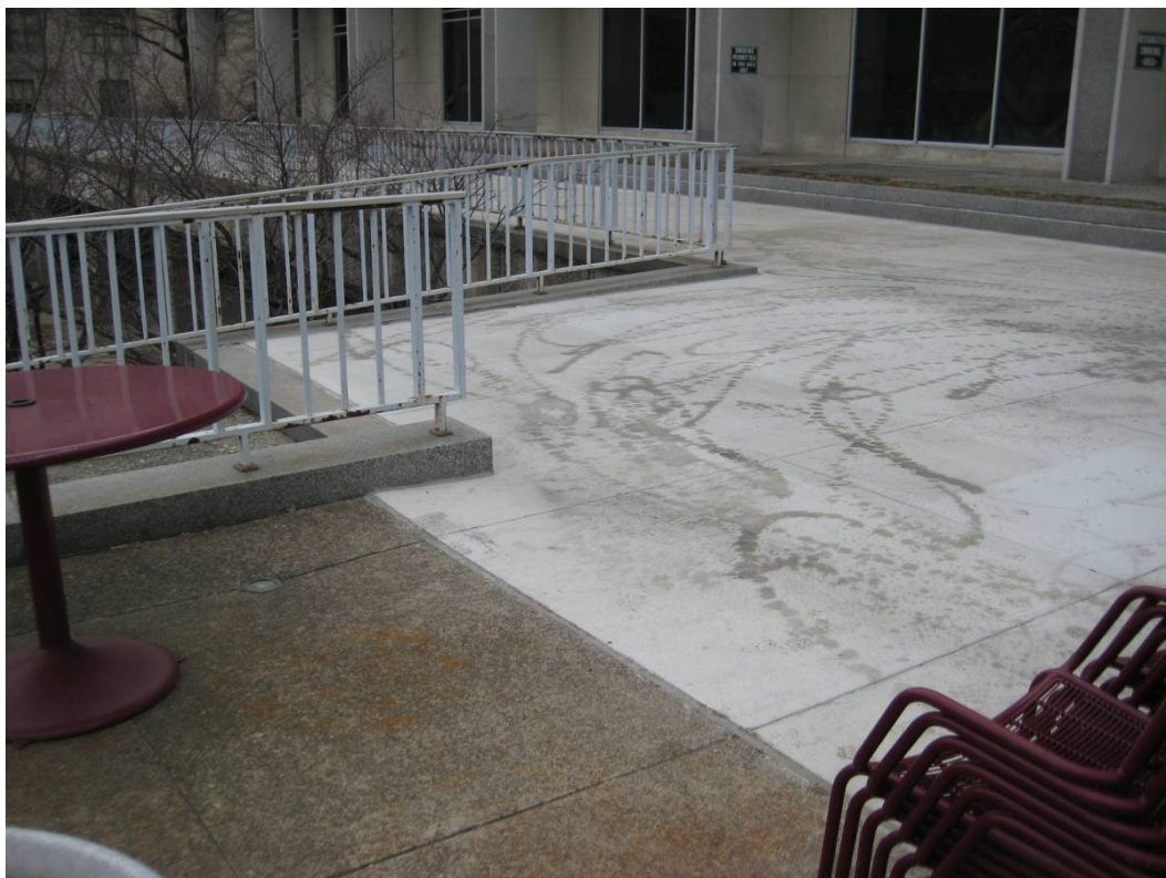
Figure 60 Plaza, looking southeast, showing replacement smooth concrete paving panels
