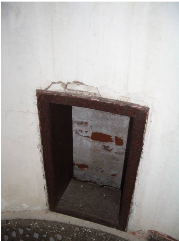
4 5 6 OI-T-05: Tower metal framed access opening (Source: A&A IMGP3228)
