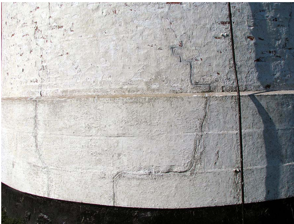
OI-T-16: Foundation and wall cracks (Source: Martin/Martin)
