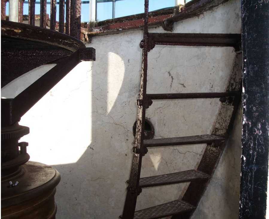
OI-T-11: Lantern with ladder to access lantern walkway (Source: A&A IMGP3210)
