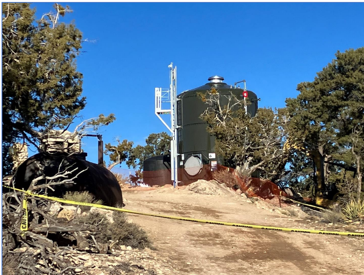
Looking Northeast from service road toward new tank with ladder and platform.
