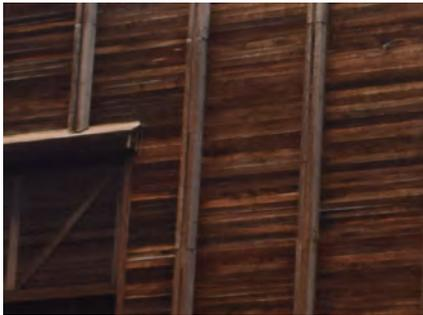
**Figure 5-43.** Natural wood siding, Filene Center (QE, 2020).
