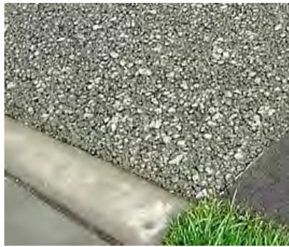
**Figure 5-15.** Permeable concrete (The Concrete Network).
