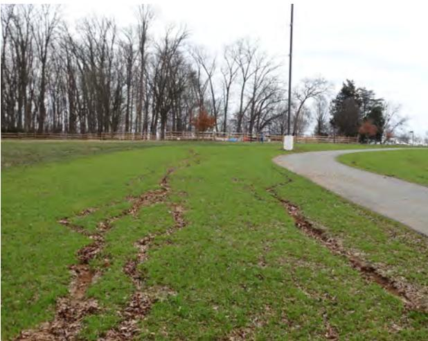
**Figure 3-110.** Erosion damage on Gil's Hill (QE, 2020).
