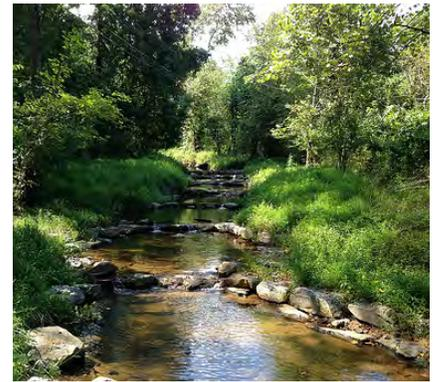
**Figure 5-6.** Step pools are constructed in the stream channel to recreate natural channel morphology. As flow moves over the step, energy is dissipated into the pool (source: Montgomery County, MD "Stream Restoration Techniques").
