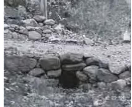
**Figure 5-33.** Rock trail culvert (USFS).
