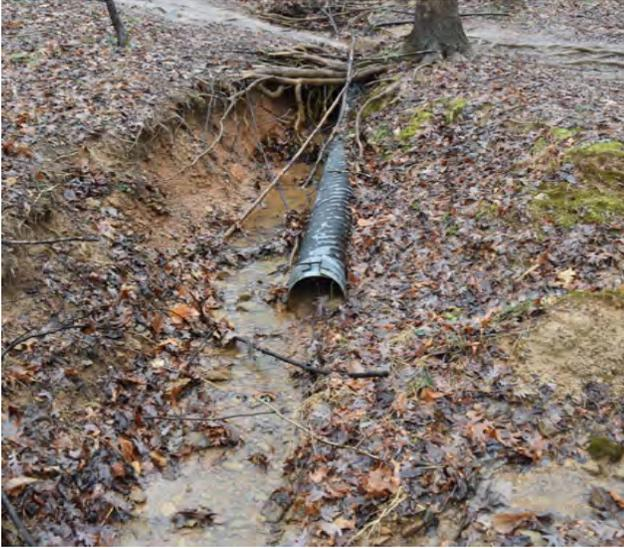
**Figure 3-167.** Slope washout near east boundary (QE, 2020).
