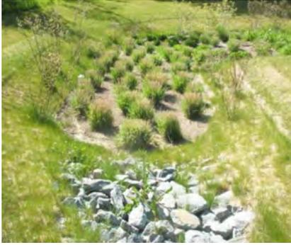
**Figure 5-11.** Bioretention area (Chesapeake Stormwater Network).
