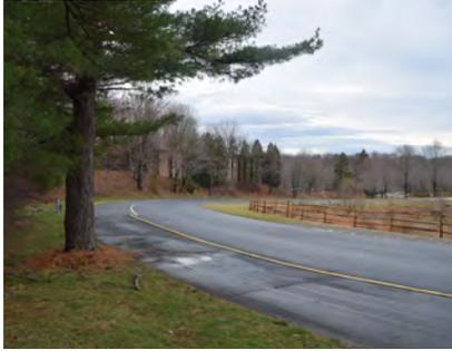
**Figure 5-19.** Two-lane asphalt road without curb (QE, 2020).
