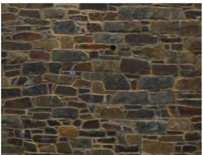
**Figure 5-51.** Squared mortared stone, Tunnel (QE, 2020).
