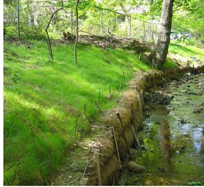
**Figure 5-2.** Fiber rolls are made of coconut fibers bundled together with biodegradable netting, and can provide temporary protection for the bank while vegetation is established (source: Montgomery County, MD "Stream Restoration Techniques").
