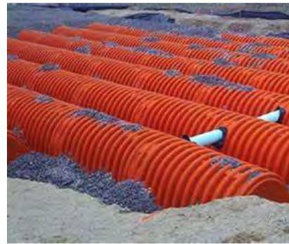
**Figure 5-16.** Sub-grade retention system (StormChambers).
