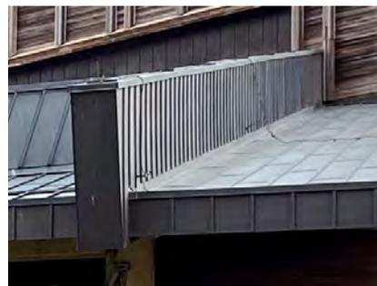
**Figure 5-53.** Standing metal seam roof, Filene Center (QE, 2020).
