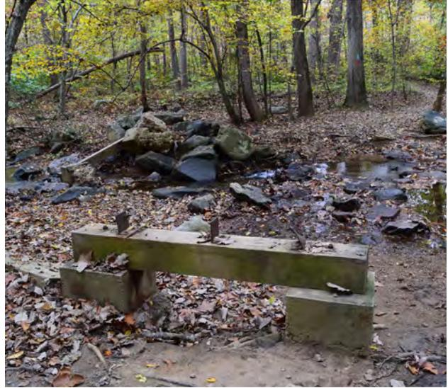
**Figure 3-168.** Washed out bridge over Old Courthouse Spring Branch (QE, 2020).
