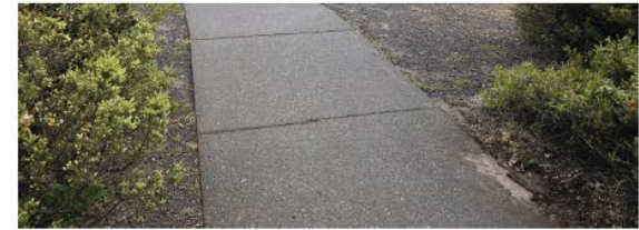
CONCRETE PAVEMENT - EXPOSED AGGREGATE CONCRETE FOOTPRINT OF JAGGAR MUSEUM WILL MATCH EXISTING PEDESTRIAN PAVEMENT ON SITE
