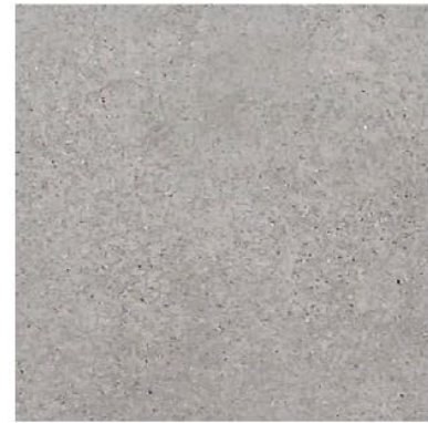
EXPOSED CONCRETE FLOOR FINISH
