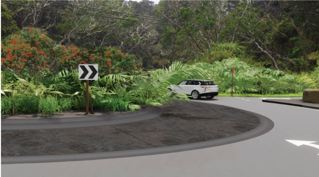
TRUCK APRON - STAMPED CONCRETE
