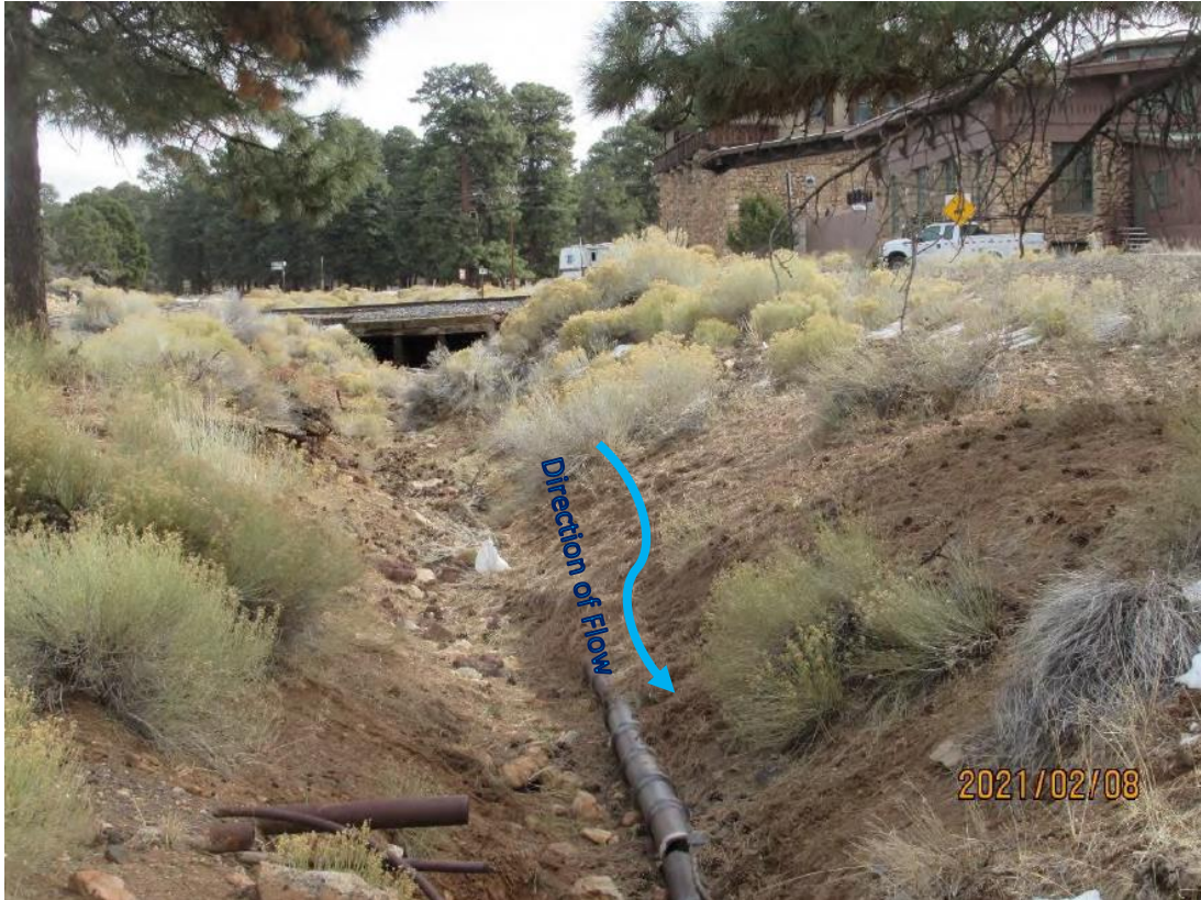
View east showing Bright Angel Wash and wooden box culvert.
