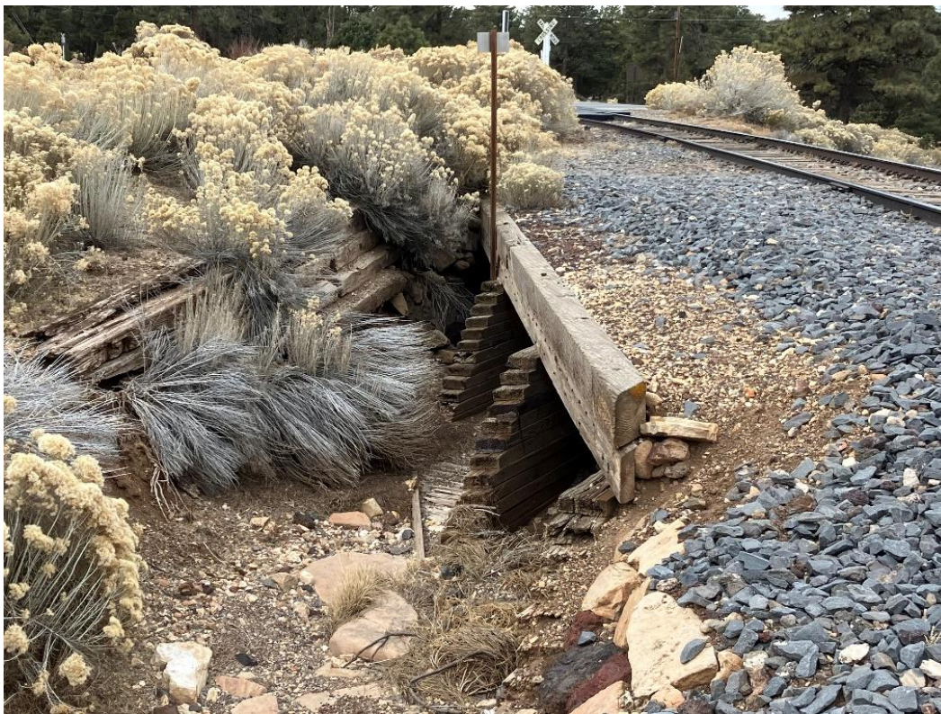
East side of wooden ballast bridge, looking southwest
