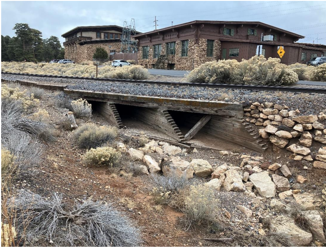
Figure 3. Existing Wooden Box Culvert
