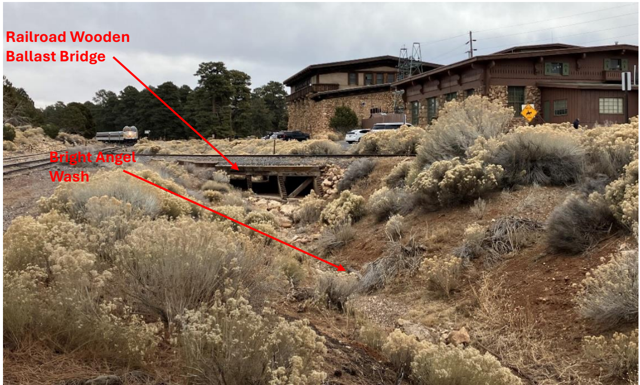
Bright Angel Wash on the west side of wooden ballast bridge, looking east (January 3, 2024)
