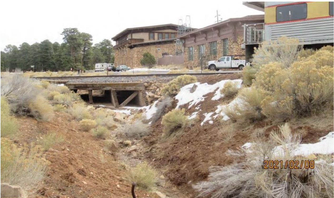
View east showing Bright Angel Wash and the railroad crossing proposed for replacement. The Powerhouse building is visible on the right side of the photo (January 8, 2021).
