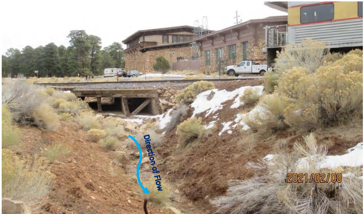
View east showing Bright Angel Wash and the railroad crossing proposed for replacement. The Powerhouse building is visible on the right side of the photo (January 8, 2021).
