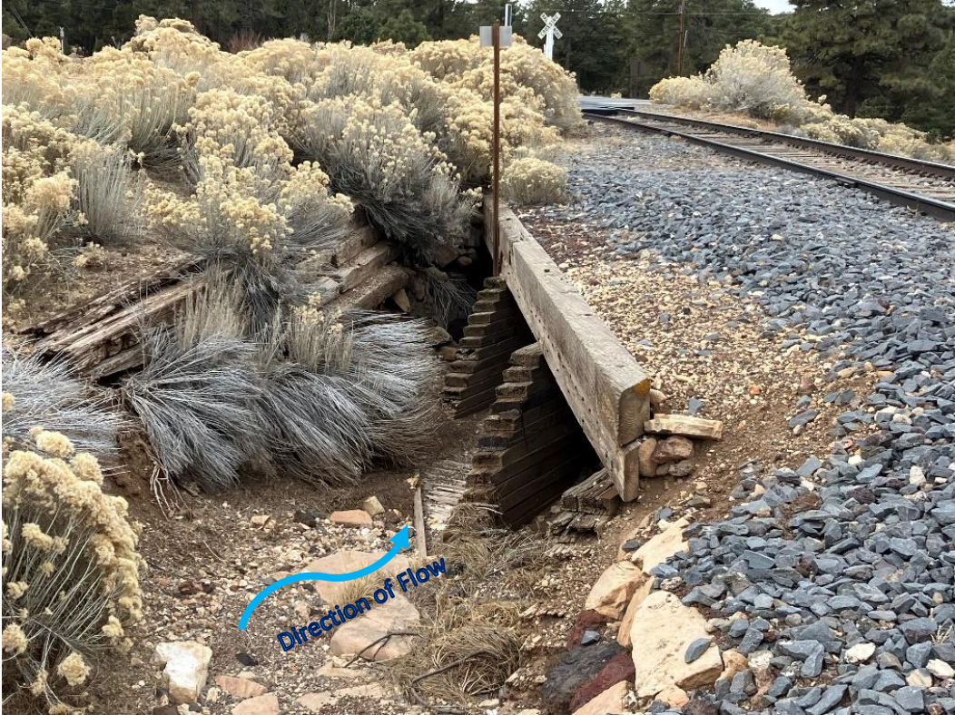
East side of wooden box culvert, looking southwest
