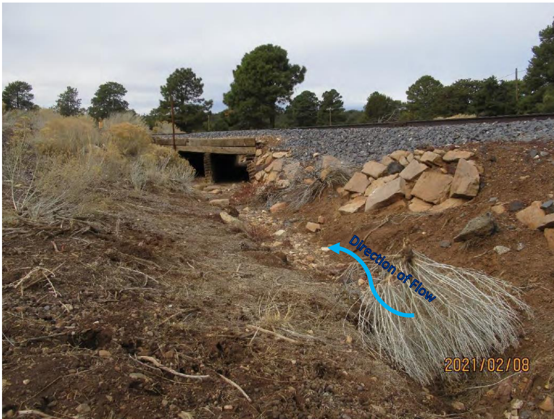
View west showing Bright Angel Wash and wooden box culvert.
