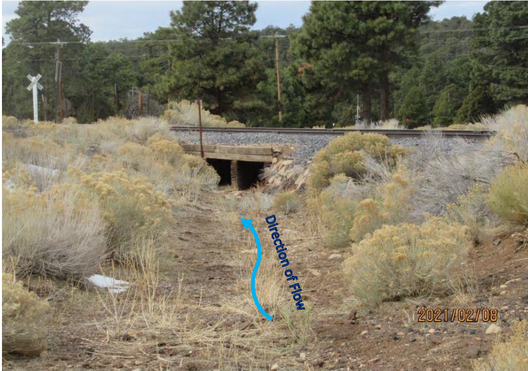
View west showing Bright Angel Wash and wooden box culvert.
