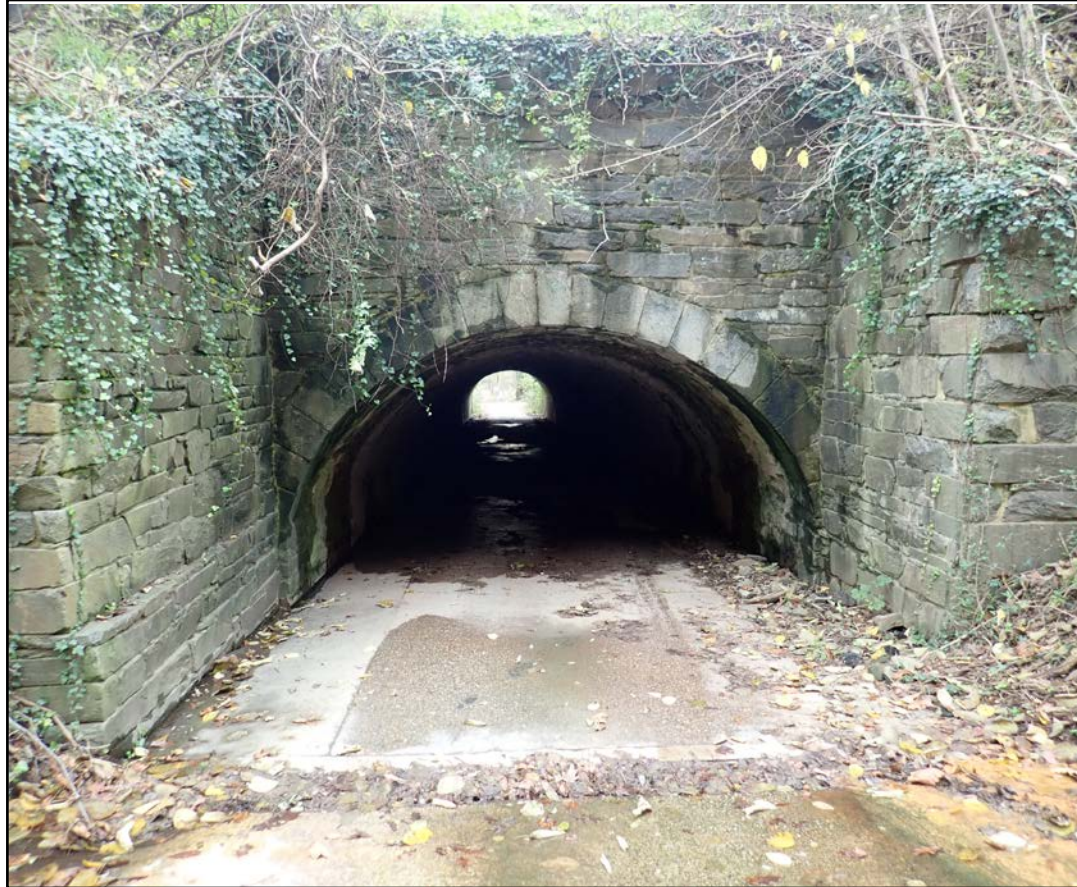
11 Road culvert (tunnel) entrance from east approach (height clearance ~7 feet)
