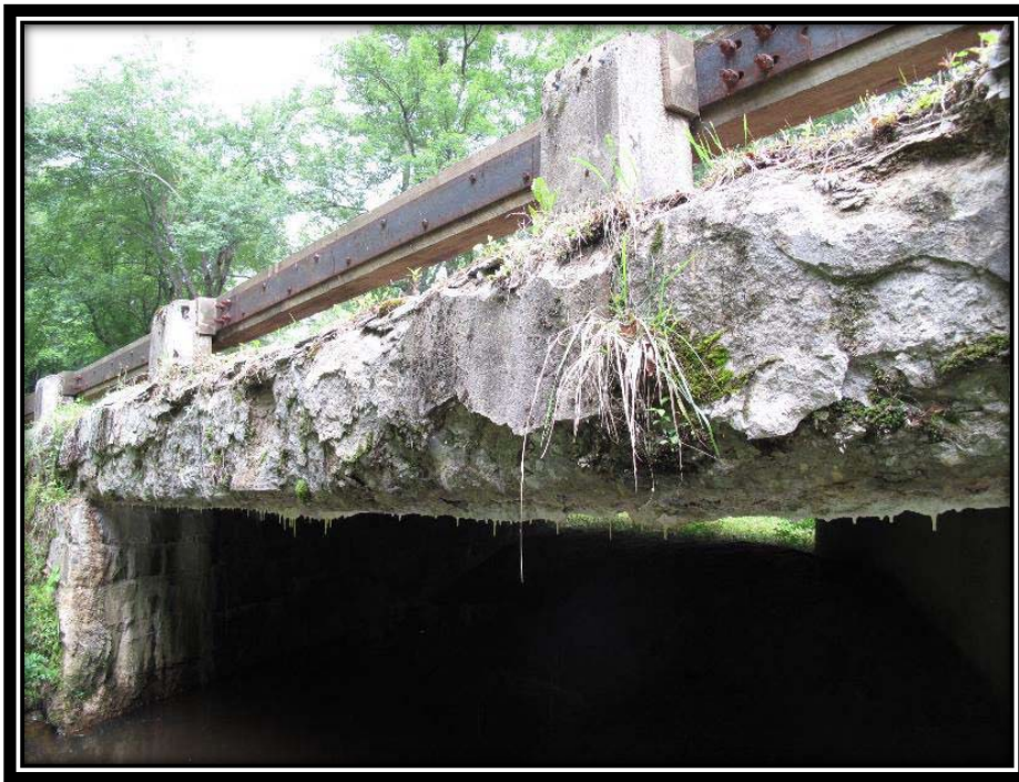
Exhibit 1: Big Pine Creek Bridge #3, Structure. 5140-077P – Side view of bridge degradation
