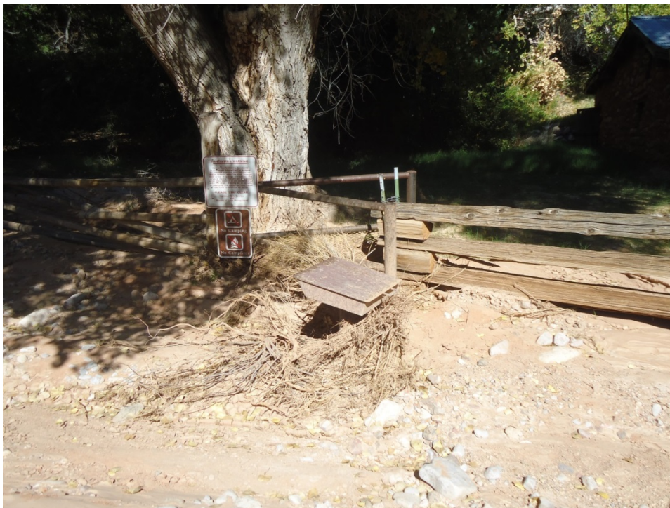
Figure F-5. Post 2014 flood. Note the bottom rail is completely buried in sediment. The trail register, when opened, was full of fine silt.
