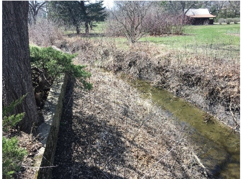
PHOTOGRAPH 6. LIMESTONE RETAINING WALL ADJACENT TO DOWNEY STREET BRIDGE.
