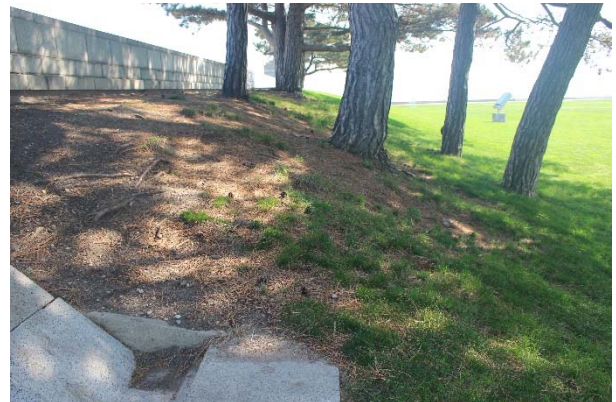
Figure 2-4: Area of erosion of the earthen berm under the Austrian pines. CHG
