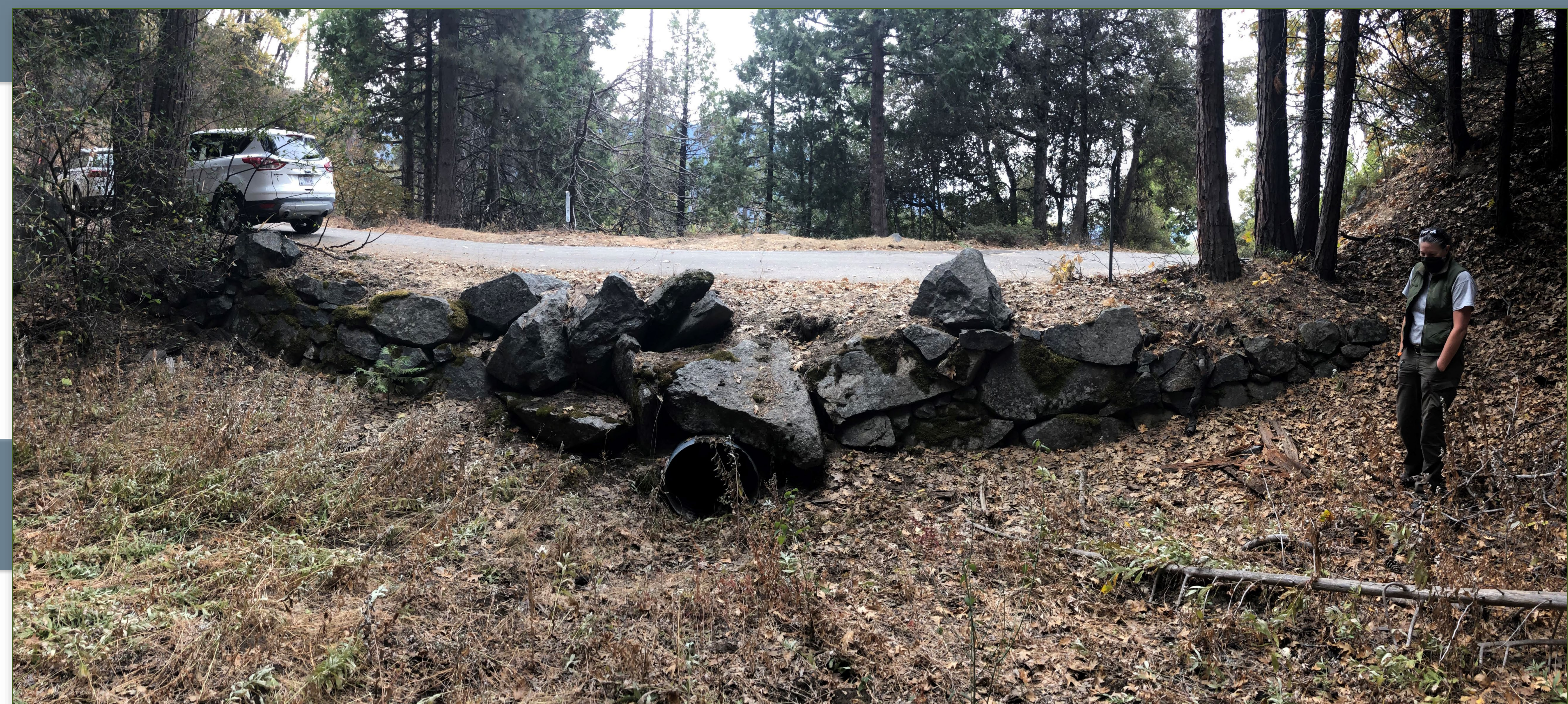
Photo: Image of rock headwall and culvert that have partially failed. Lower section of Mineral King Road. NPS Photo.
