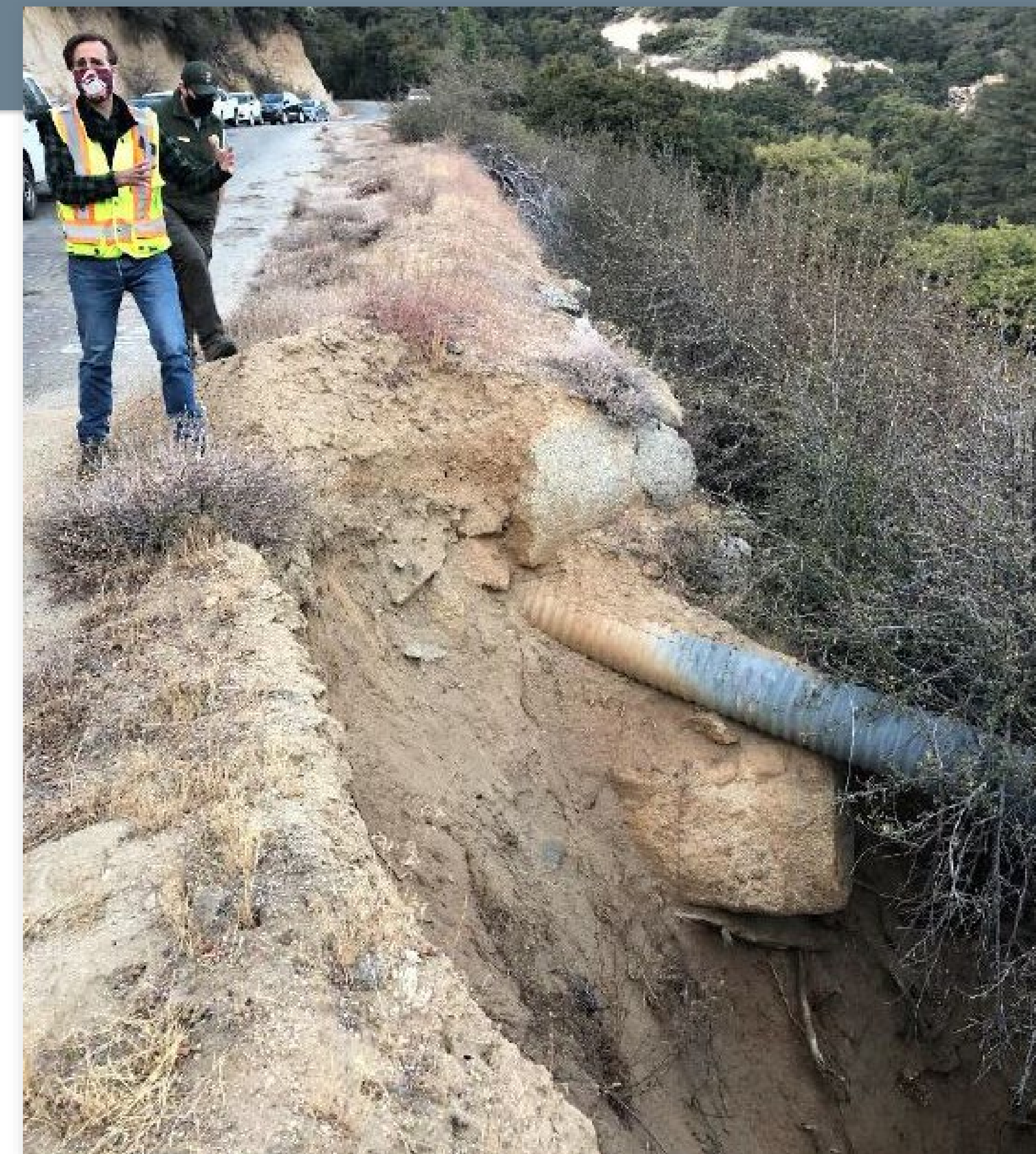
Photo: Project Planners and Engineers stand above an eroded slope along the lower section of Mineral King Road. Culvert extends out beyond roadway. NPS Photo.
