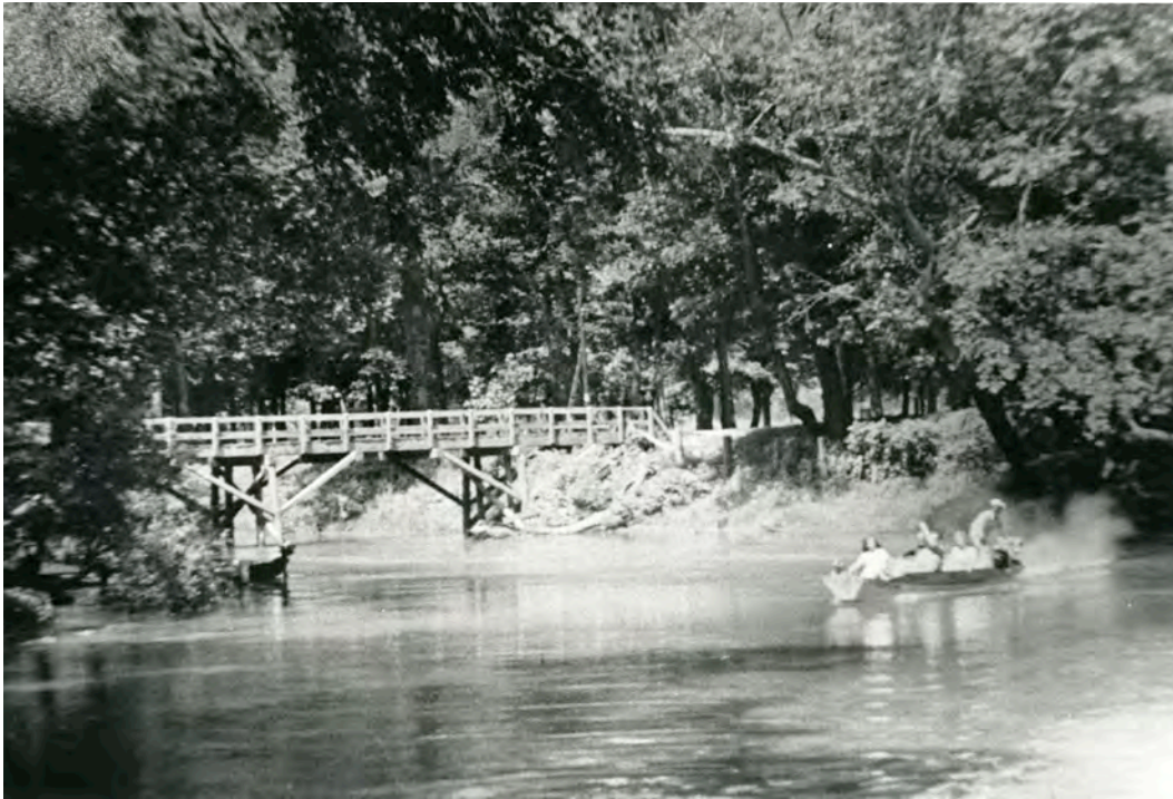
Figure 3-134. Big Spring Branch Vehicular Bridge, note diagonal struts, Circa 1940. (OZAR Archives)
