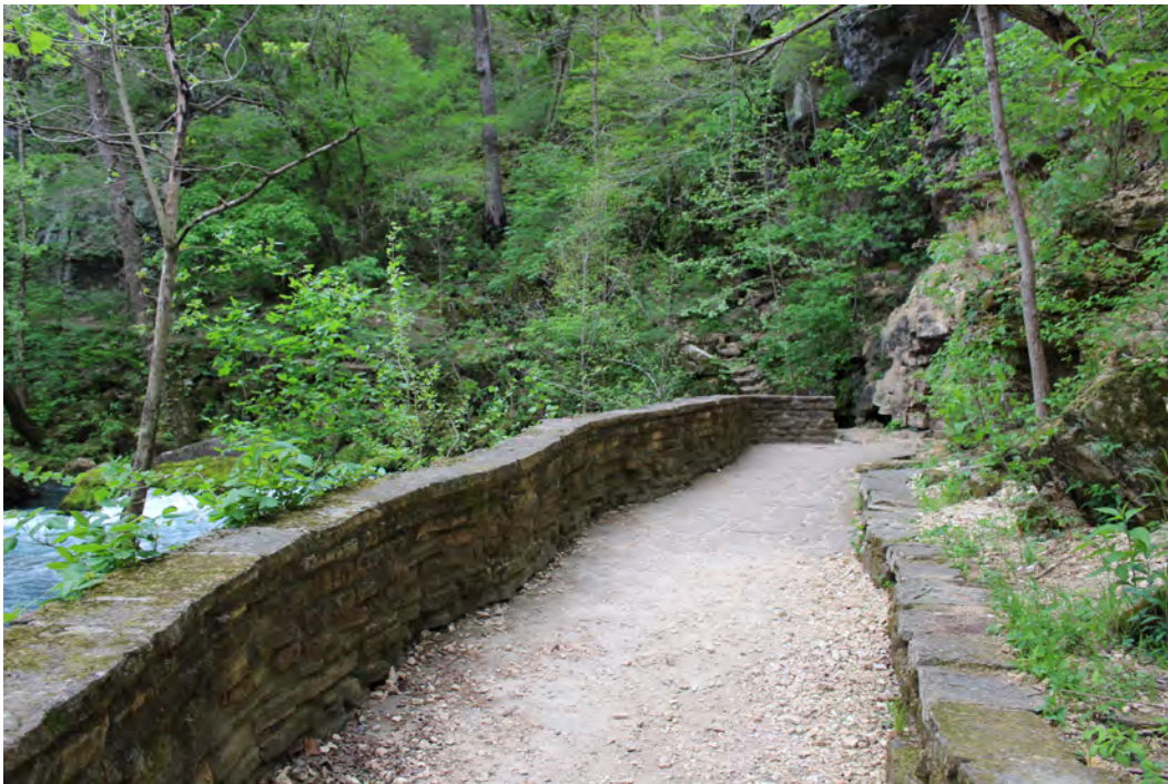
Figure 3-137. The trail to the spring from the parking area has been modified since the period of significance with new stone surfacing and retaining walls. (Mundus Bishop 2016)
