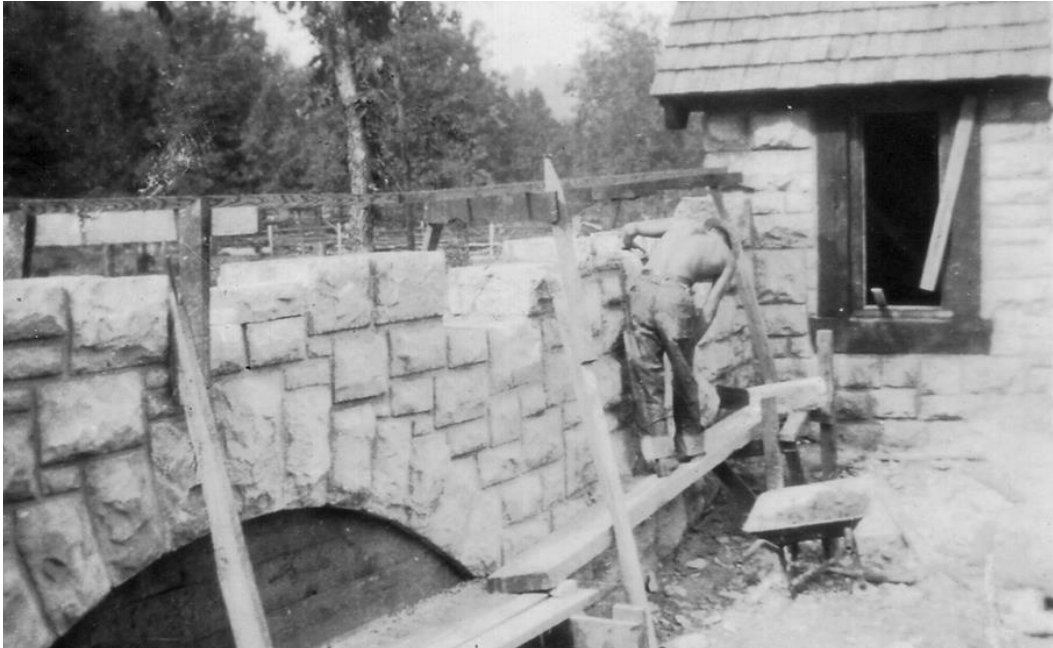
Figure 3-59. East Entrance Portal Wall (HS-432A) arch over ditch during construction, 1936. (OZAR Archives)
