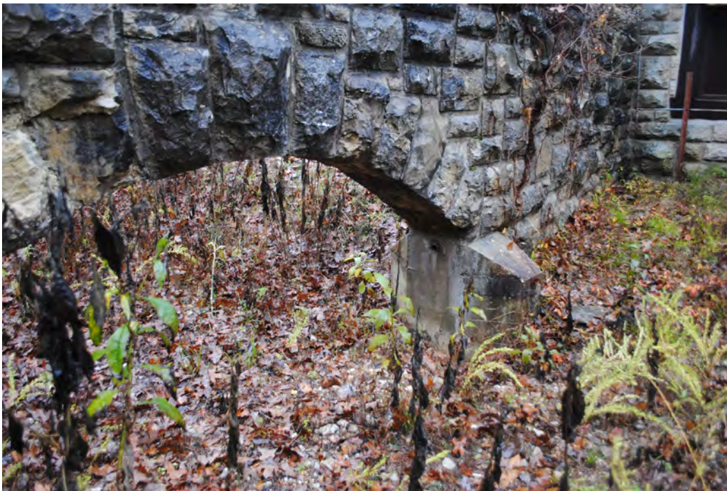
Figure 3-60. East Entrance Portal Wall (HS-432A) arch over ditch. (Mundus Bishop 2015)
