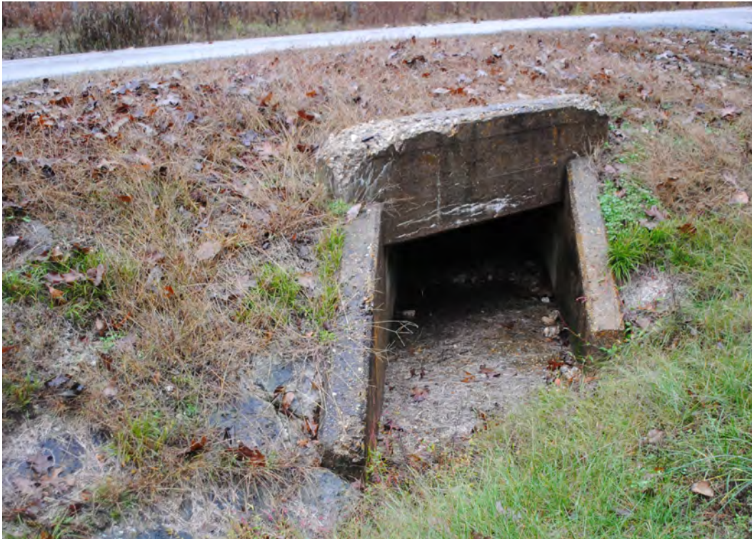
Figure 3-51. The stone and concrete culvert extends under Peavine Road / State Highway 103. (Mundus Bishop 2015)
