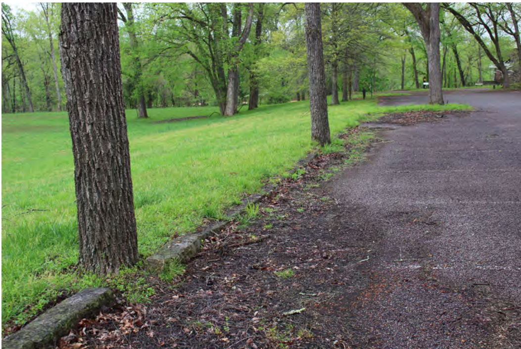
Figure 3-30. The CCC stone retaining curb at the Main Parking Area (HS-714) is in fair to poor condition. (Mundus Bishop 2016)
