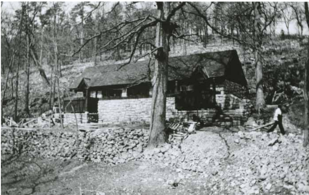
Figure 2-60. The CCC built the Latrine (HS-423) with exposed timber framing and irregular coursed cut stone walls. A stone retaining wall and abutments were dry laid against the embankment, date unknown. (OZAR Archives)
