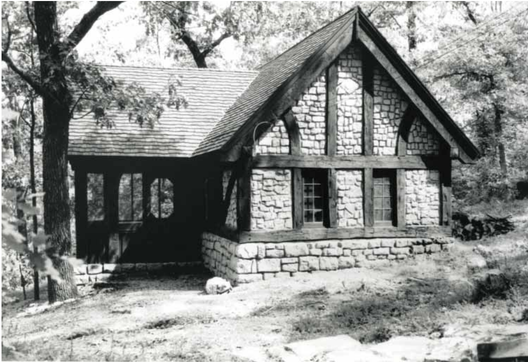
Figure 2-46. Cabin #402 (HS-402) (shown) and Cabin #403 (HS-403) were constructed with exposed timber framing and irregular coursed cut stone walls. Both are 'type A' cabins, date unknown. (OZAR Archives)
