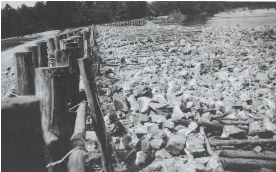
Figure 2-32. The rock fill of the Big Spring Stone Dikes (HS-711) was built with an apron of rip-rap on each side of the work to prevent scouring and undermining, date unknown. (OZAR Archives)
