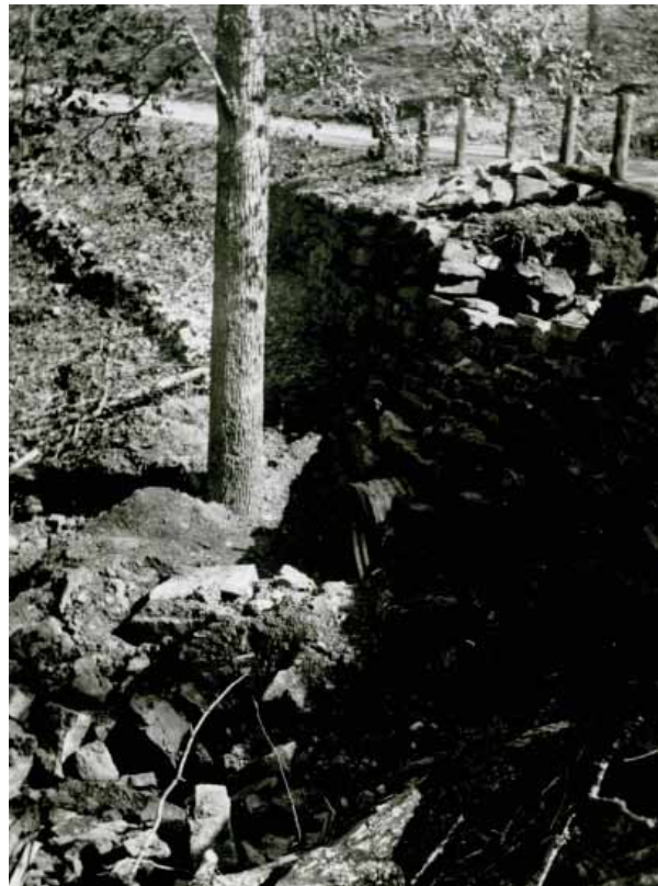
Figure 2-41. The CCC built stone culverts to direct water under roads, date unknown. (OZAR Archives)
