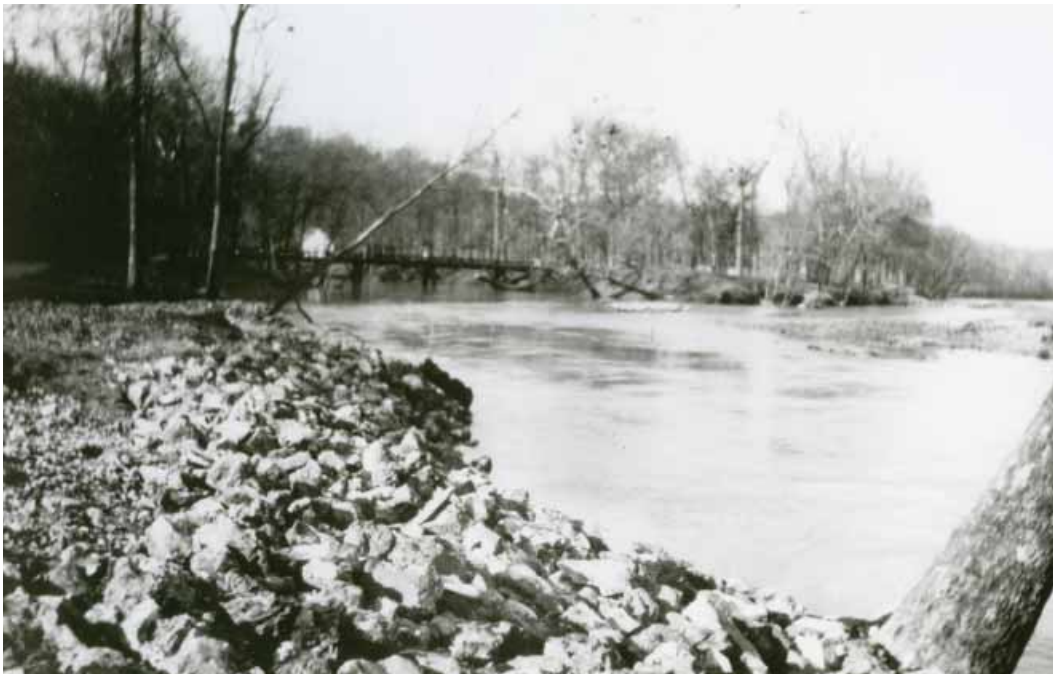
Figure 2-39. The CCC stabilized the drainage channels and stream edges with stone, date unknown. (OZAR Archives)
