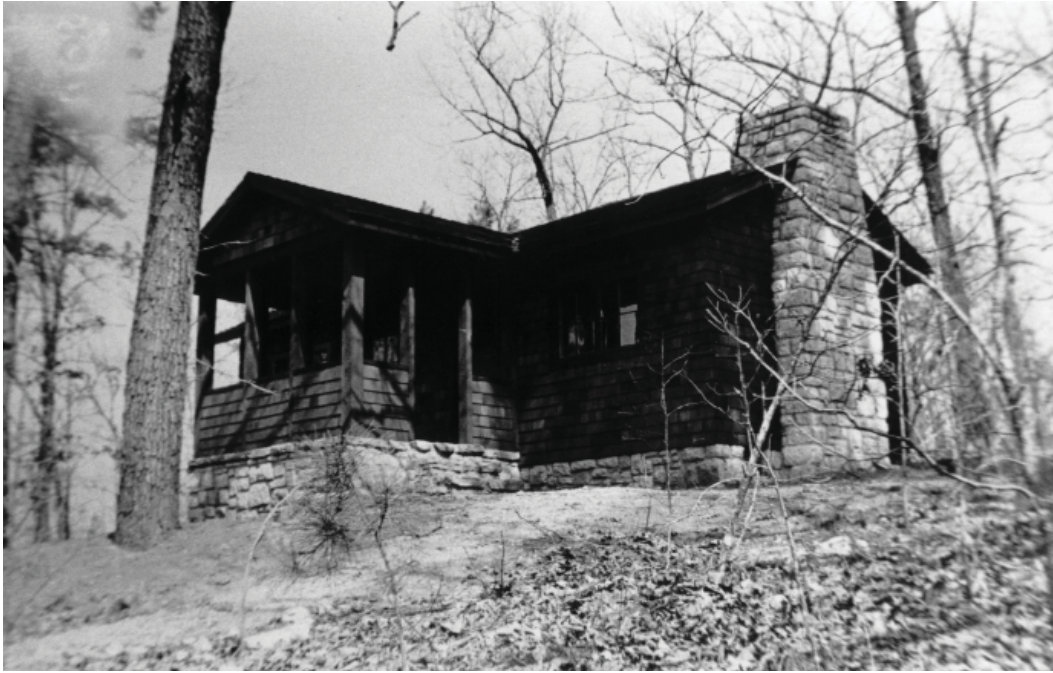
Figure 2-53. Cabins #406 (HS-406), #407 (HS-407), and #408 (HS-408) were relocated and remodeled with new screen porch entries and exterior stone chimneys, date unknown. (OZAR Archives)
