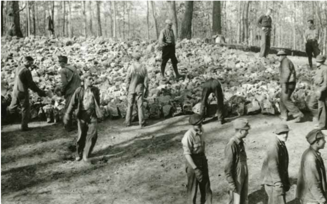
Figure 2-40. The CCC stabilized steep slopes with rock outcropping from the quarry, date unknown. (OZAR Archives)
