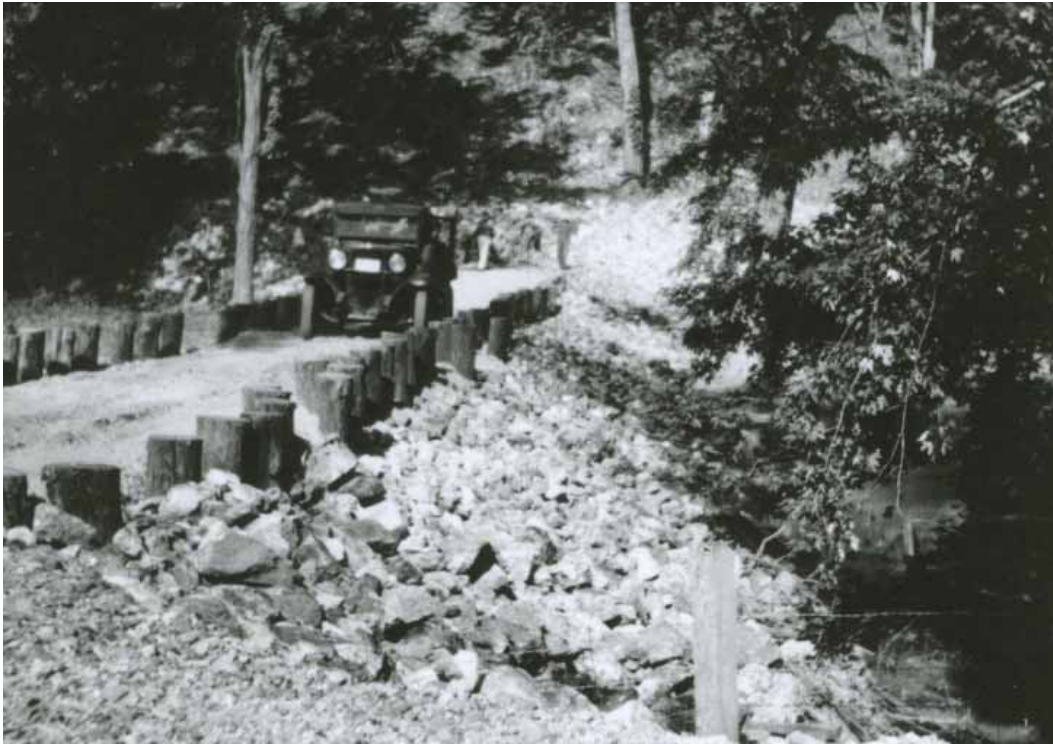
Figure 2-31. The Big Spring Stone Dikes (HS-711), constructed of stone and oak timber helped prevent the Current River from flooding Big Spring, date unknown. (OZAR Archives)
